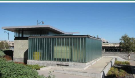
Updated pump stations and infrastructure
