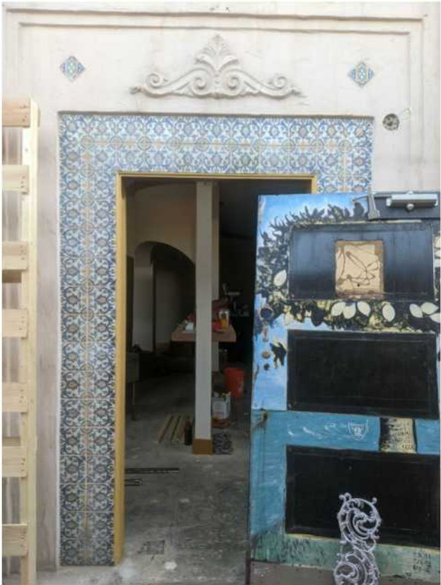
RESTORED FRONT ENTRY AND DOOR
