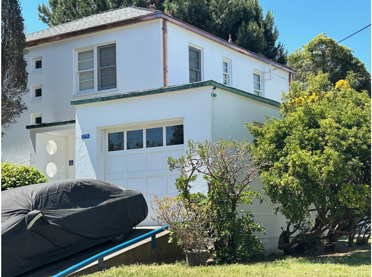
NEWLY REPLACED COPPER GUTTERS / DOWNSPOUTS ON UPPER ROOF WITH ORIGINAL COPPER GUTTERS ON LOWER ROOFS
