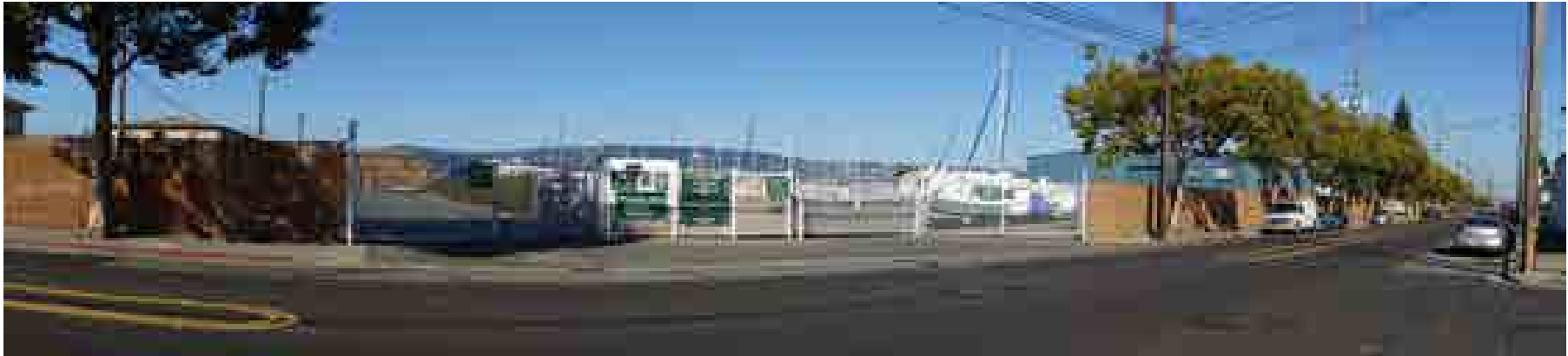
Photo 1a: View of existing Alameda Marina facility looking northeast from intersection of Clement Avenue and Stanford Street.
