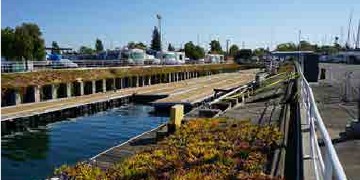
Photo 6: View looking south of existing graving dock.
