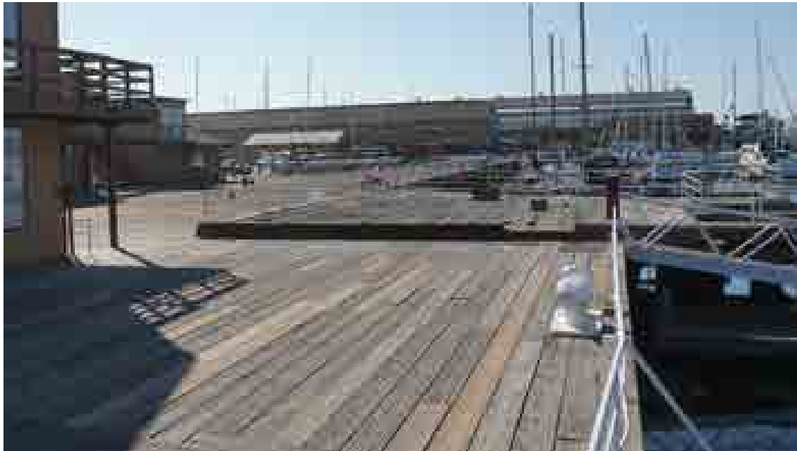
Photo 5a: View looking northwest of existing wharf facilities within Alameda Marina.
