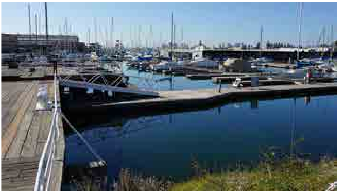
Photo 5b: View looking northwest of existing wharf and dock facilities within Alameda Marina.
