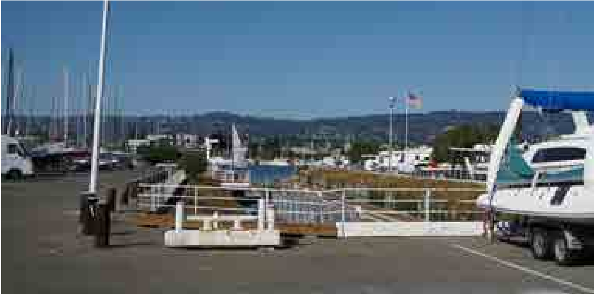
Photo 7: View looking north of existing graving dock facility.
