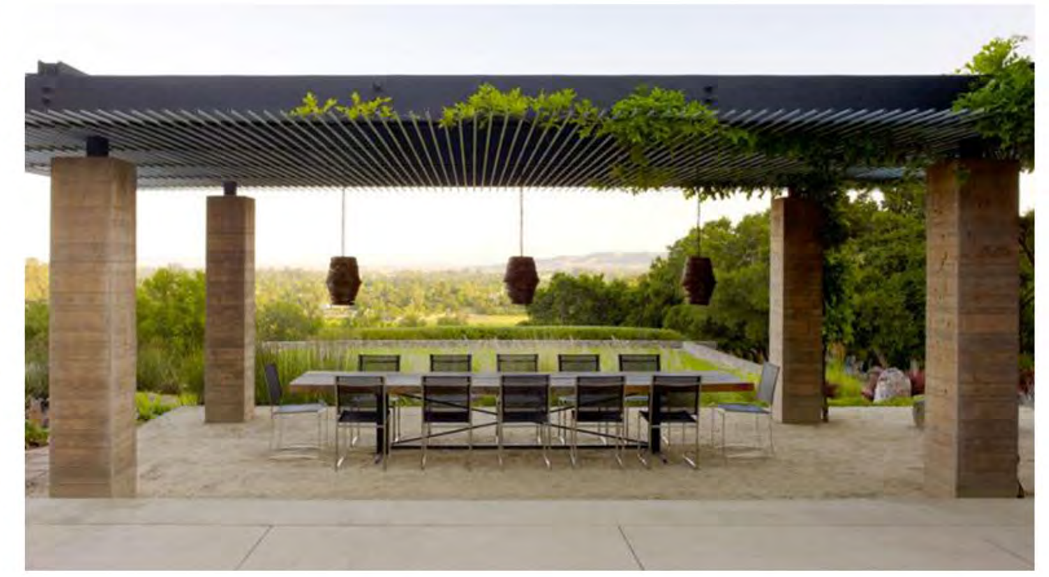
SHADE STRUCTURE, Precast Columns with Wood Trellis
