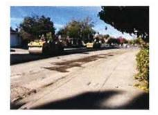
lift for the new street section. Work scope also included sidewalk repair, curb ramp installations, adjustment of existing utility covers, striping, signage and a section of fiber optics conduit with pull boxes.
