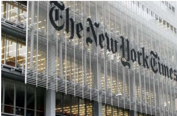
This screen/grille on the New York Times Building doubles as a sign. It permits light into the building but presents as a solid object to birds.
