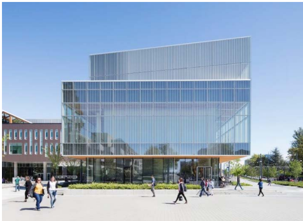
Glass facade with vertical frit pattern, University of British Columbia Library.
