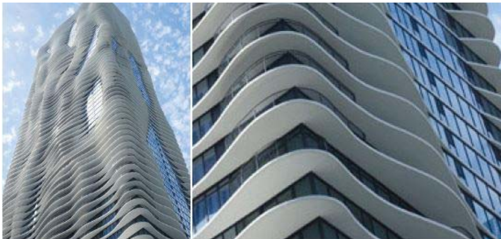
Louvres, Aqua Tower, Chicago
