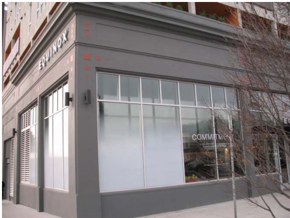
Translucent glass on portion of the storefront in a recently constructed mixed-use building, Berkeley.
