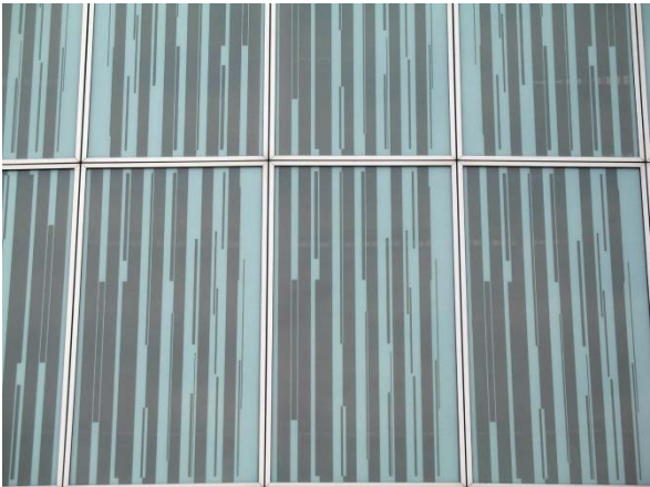
Close-up of fritted glass on Cathedral of Christ the Light.
