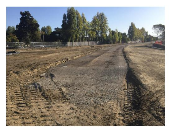
Photo 19: View of AB Layer on top of compacted and sealed Consolidation Area
