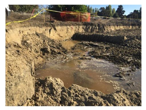
Photo 6: Water Table Encountered at Overexcavated Section from Area
