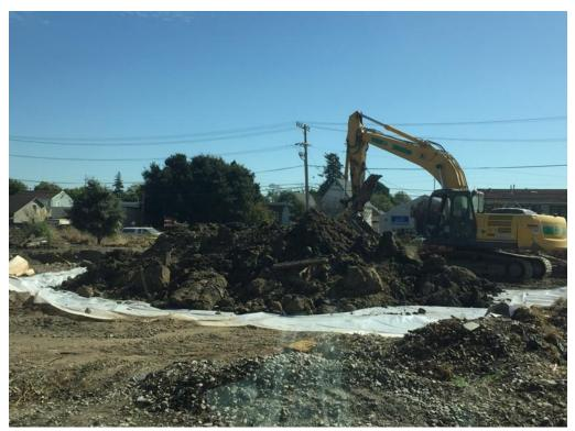
Photo 12: Office Stockpiling of Non-Saturated Impacted Soil from Excavation Area C on Visqueen for Offhaul
