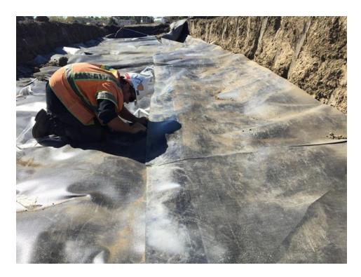
Photo 17: Sealing of HDPE Liner with Adhesive
