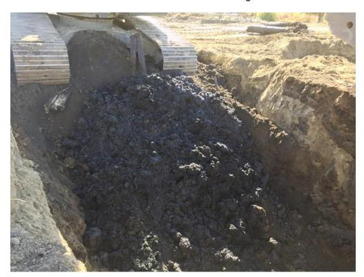
Photo 10: Impacted Patch of Soil and Debris from under Railroad Platforms in Excavation Area C Prior to Removal
