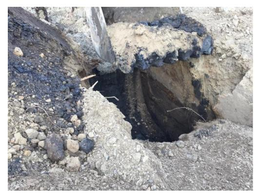
Photo 11: Removal of Patch of Impacted Soil and Debris from Northeast Arm of Excavation Area C
