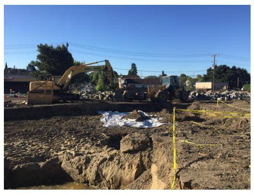
Photo 7: Removal of Concrete Sump from the South Corner of Excavation Area B after Overexcavation
