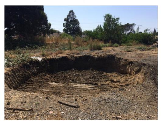
Photo 14: Completed Removal of Impacted Soil from East Lead Impacted Area
