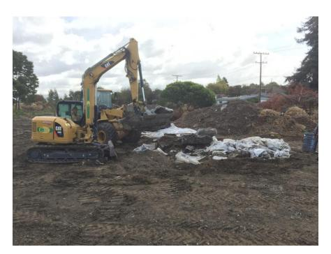
Photo 22: Concrete Sump Pieces Placed in Loader to Move to Truck for Transportation and Disposal
