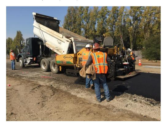
Photo 20: Paving of Asphalt Layer of Cap
