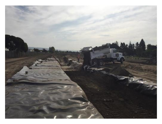
Photo 15: Placement of Non-Saturated Soil into the HDPE Lined Consolidation Area
