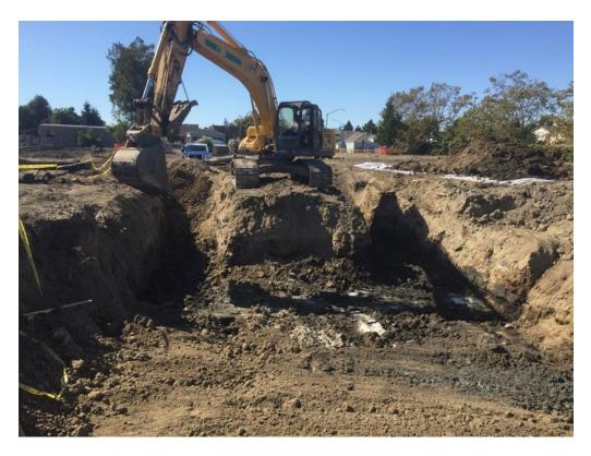
Photo 13: Near Completion of Removal of Impacted Soil from Excavation Area C
