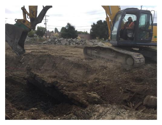
Photo 9: Railroad Platforms and Ties Encountered During the Excavation of Area C
