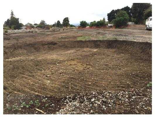
Photo 8: Completed Removal of Impacted Soil from Excavation Area D
