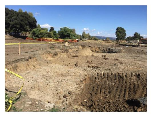
Photo 2: View of Excavation Area A Overexcavation
