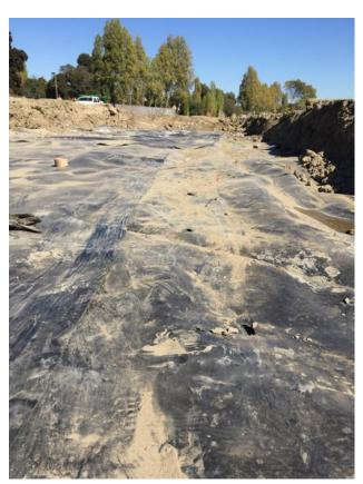
Photo 18: Sealed HDPE Lined Consolidation Area
