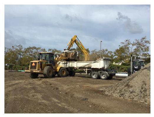
Photo 23: Loader Places Excess Impacted Soil and Visqueen Liner into Truck for Transportation and Disposal
