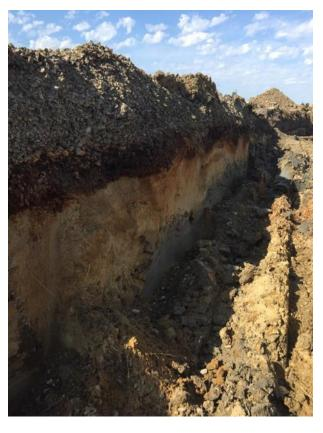
**Photo 5:** Impacted Sidewall in Excavation Area B Prior to Overexcavation
