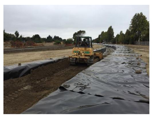
Photo 16: Compaction of Non-Saturated Impacted Soil Placed in HDPE Lined Consolidation Area
