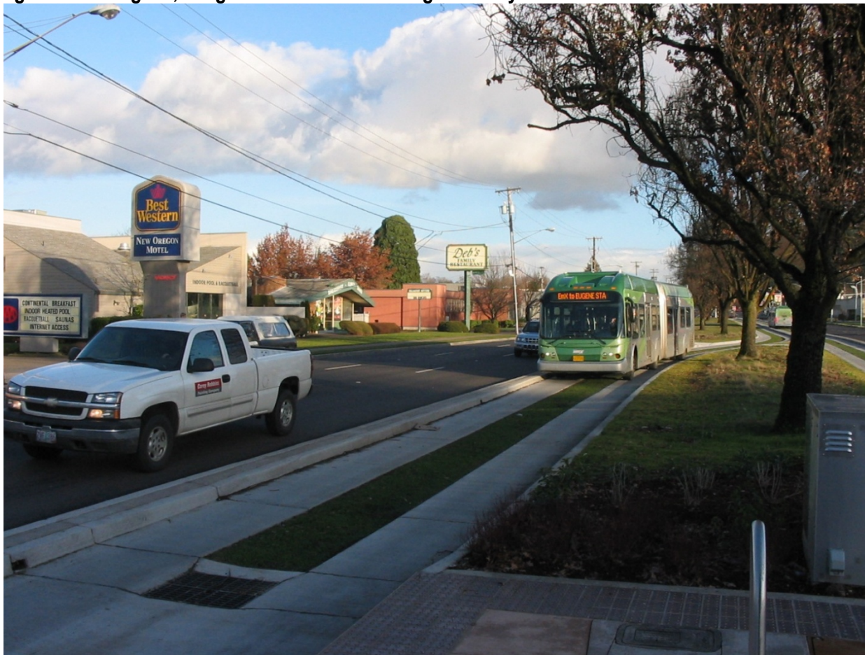
Figure 1-7 Eugene, Oregon BRT Vehicle and Right-of-Way
