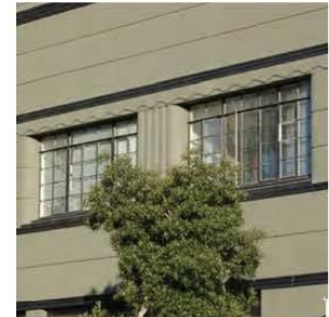
Horizontally proportioned steel sash windows with rounded window recesses.
