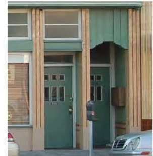
Pilasters frame building entries.
