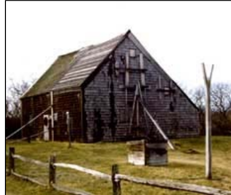
Buildings seriously damaged by storms or deterioration may need to be braced before architectural evaluations can be made. Photo: John Milner Architects. Photo: NPS files
