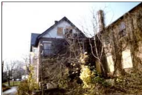
Boarding up without adequate ventilation and maintenance has accelerated deterioration of this property. Photo: NPS files.
