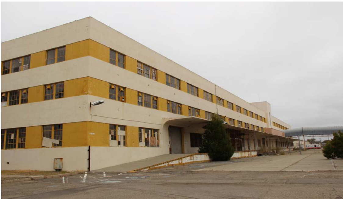
Figure 11. South façade of Building 8; view toward northeast.
