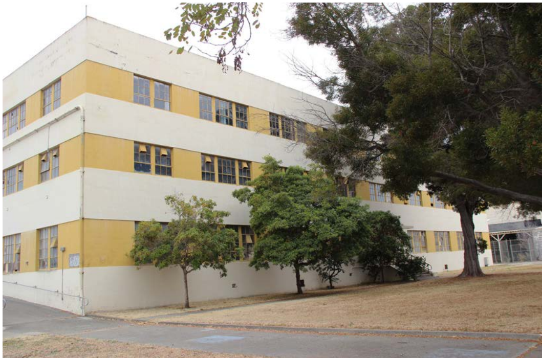
Figure 14. Detail of west façade of Building 8; view toward southeast.
