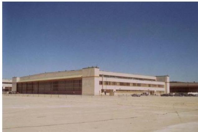
Figure 31. Building 40 (Seaplane Hangar), 2004
