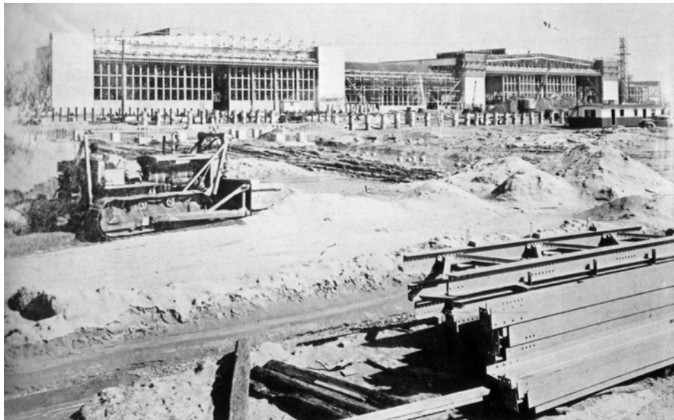
Figure 10. Building 5 under construction, April 1940. Courtesy of the National Archives Pacific Region, San Bruno
