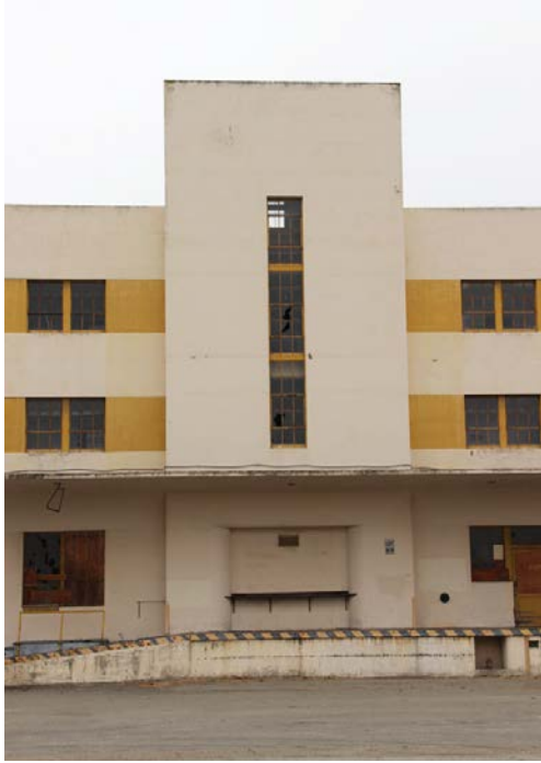
Figure 12. Tower on north façade of Building 8; view toward south.
