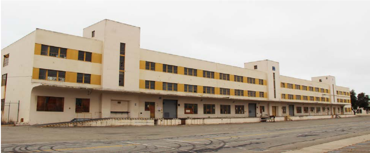
Figure 10. North façade of Building 8; view toward southwest.
