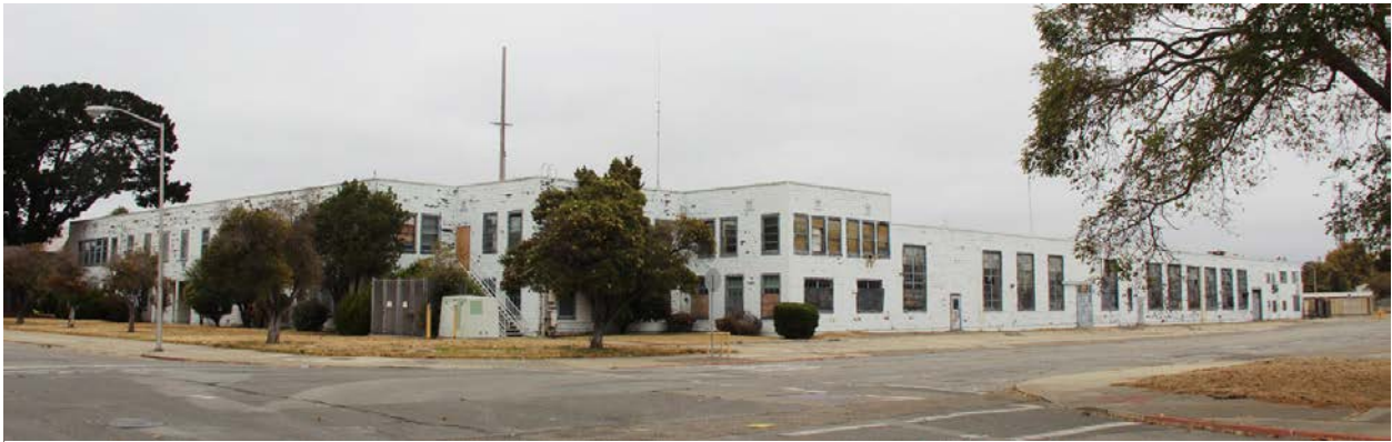
Figure 8. Building 114; view toward northeast.
