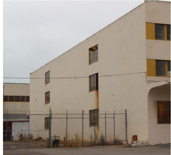
Figure 15. East façade of Building 8; view toward south.
