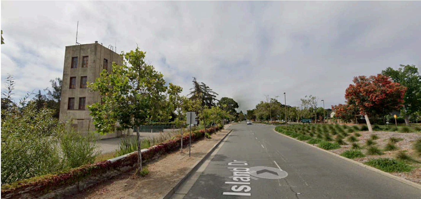
View of the North side of the tower from Island Dr.
