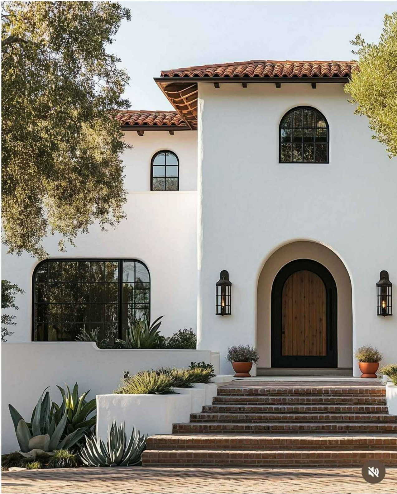
Warm White Smooth Hand Trowel Stucco / Black Clad Windows/Bullnose corners
