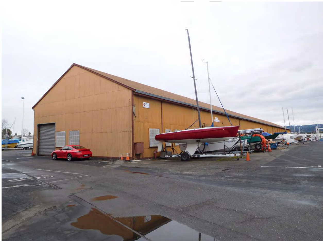
Figure 69. Building 22; south and east façades, view toward north, 2017.
