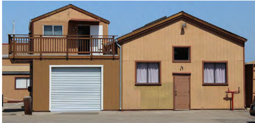
Figure 40. Building 8; east façade, view toward west, 2016.
