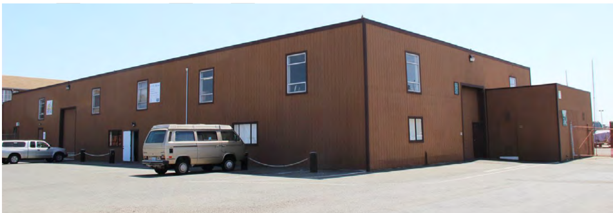
Figure 84. Building 32; south and west façades, view toward northeast, 2016.
