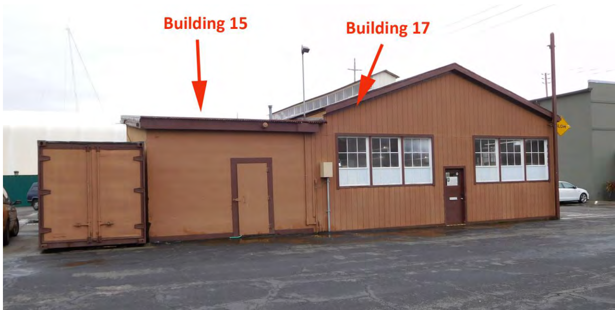
Figure 55. Buildings 15 and 17; west façade, view toward southeast, 2016.
