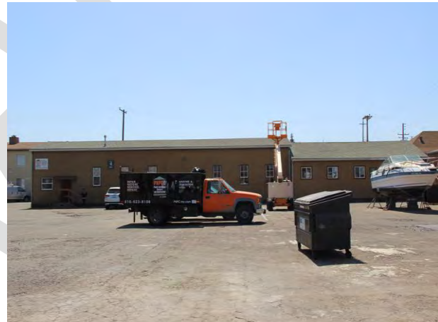
Figure 23. Small shops area showing Building 3-4 and parking lot; view toward southeast, 2016.
