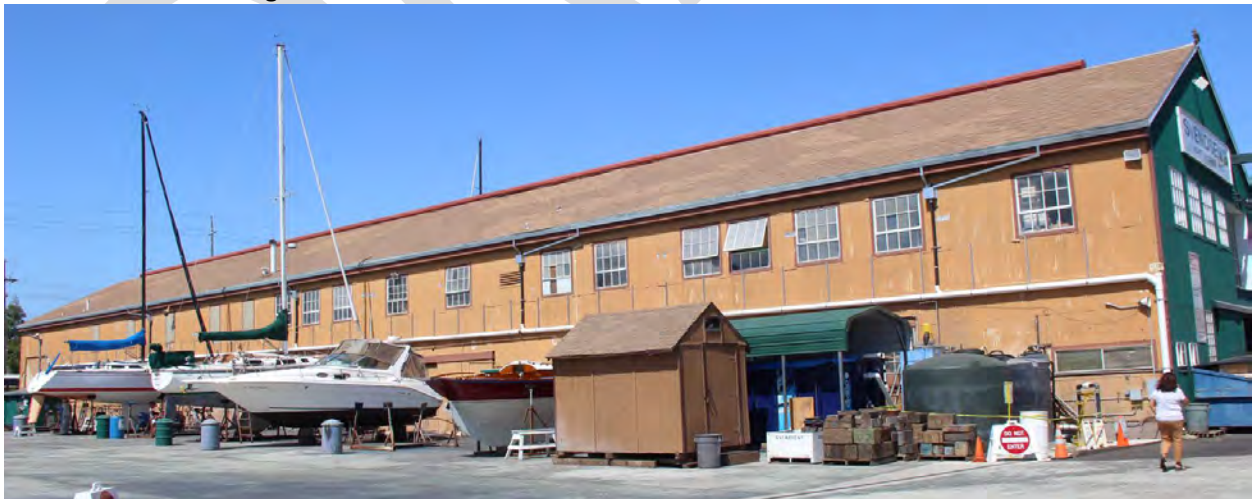
Figure 49. Building 12; east facade, view toward west, 2016.
