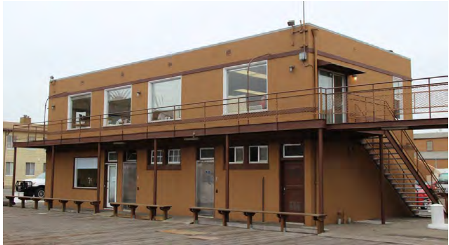
Figure 36. Building 6; north façade, view toward southeast, 2016.
