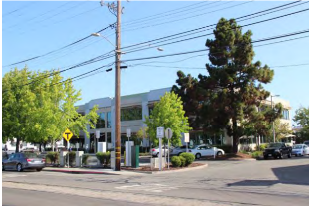
Figure 3. Alameda Power Company, 2000 Grand Street, 2016.
