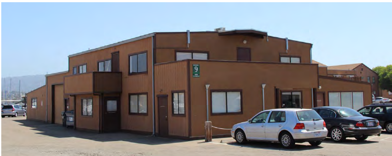
Figure 43. Building 9; south and west façades, view toward northeast, 2016.
