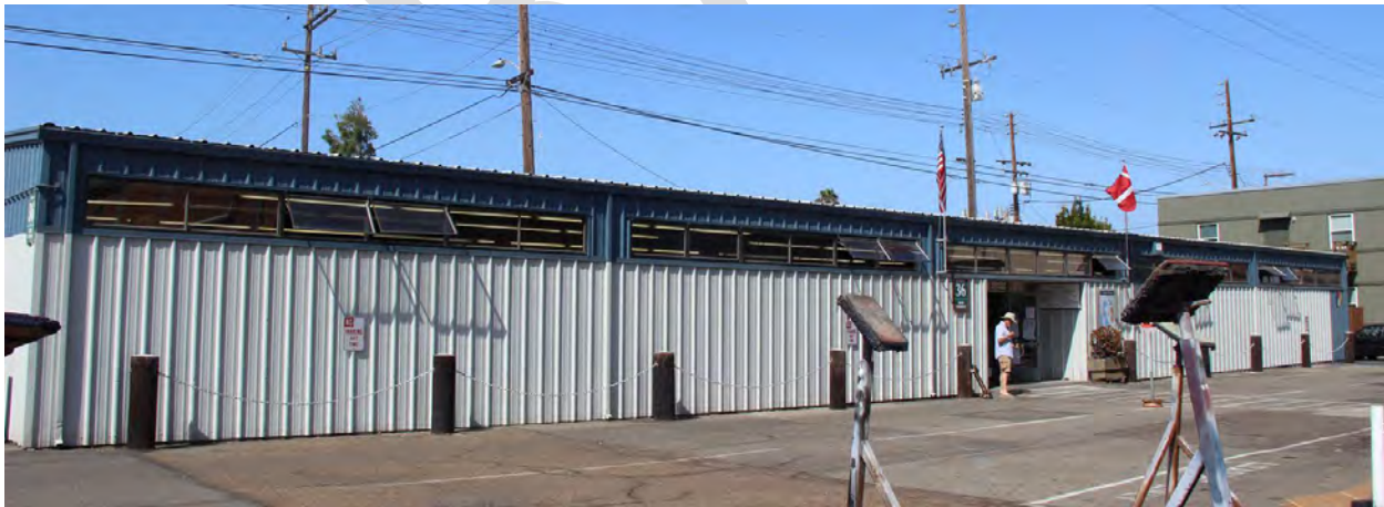
Figure 88. Building 36; view toward southwest, 2016.
