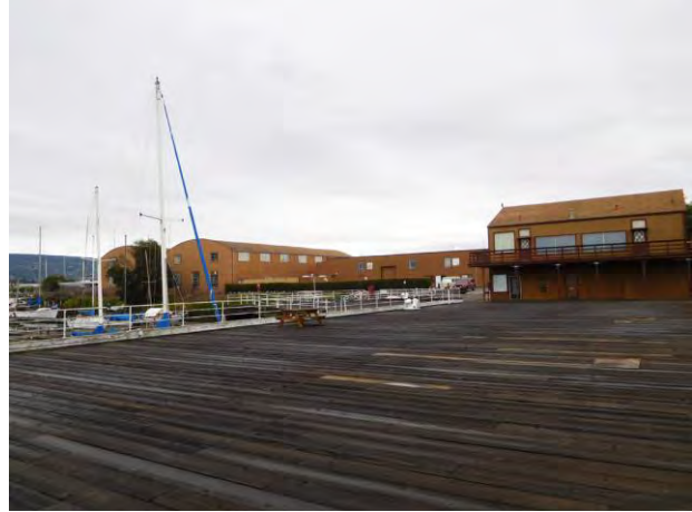
Figure 17. View of central portion of Alameda Marina property showing wharf; view toward east, 2017.
