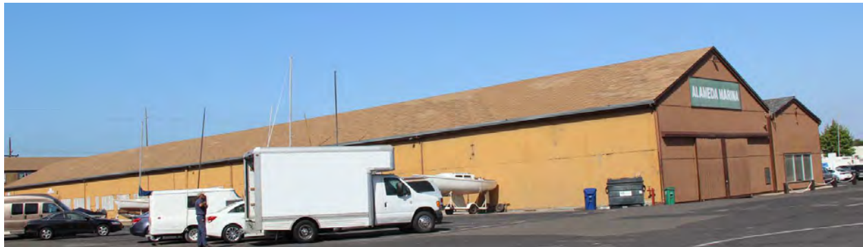
Figure 68. Building 22; east and north façades, view toward southwest, 2016.
