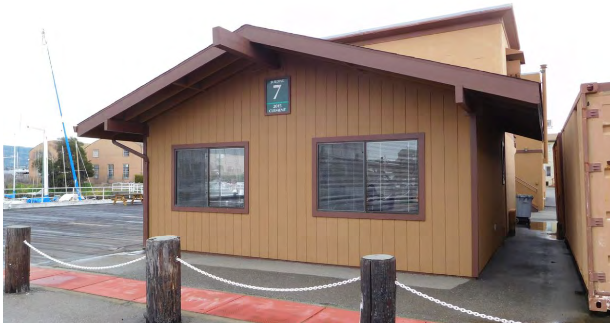
Figure 39. Building 7; west façade, view toward east, 2017.
