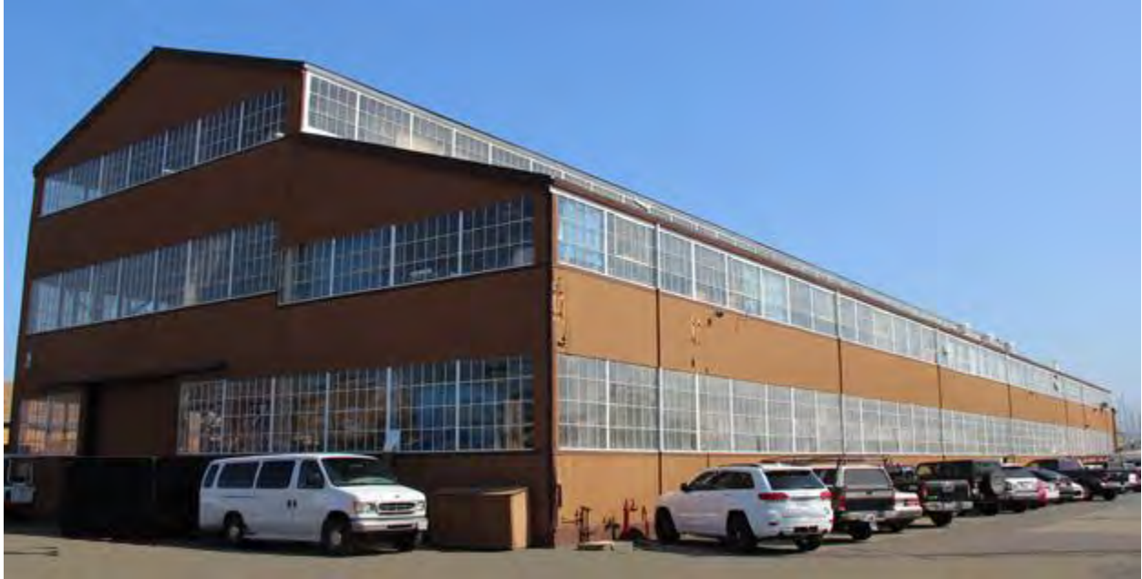
Figure 61. Building 19; view toward northwest, 2016.
