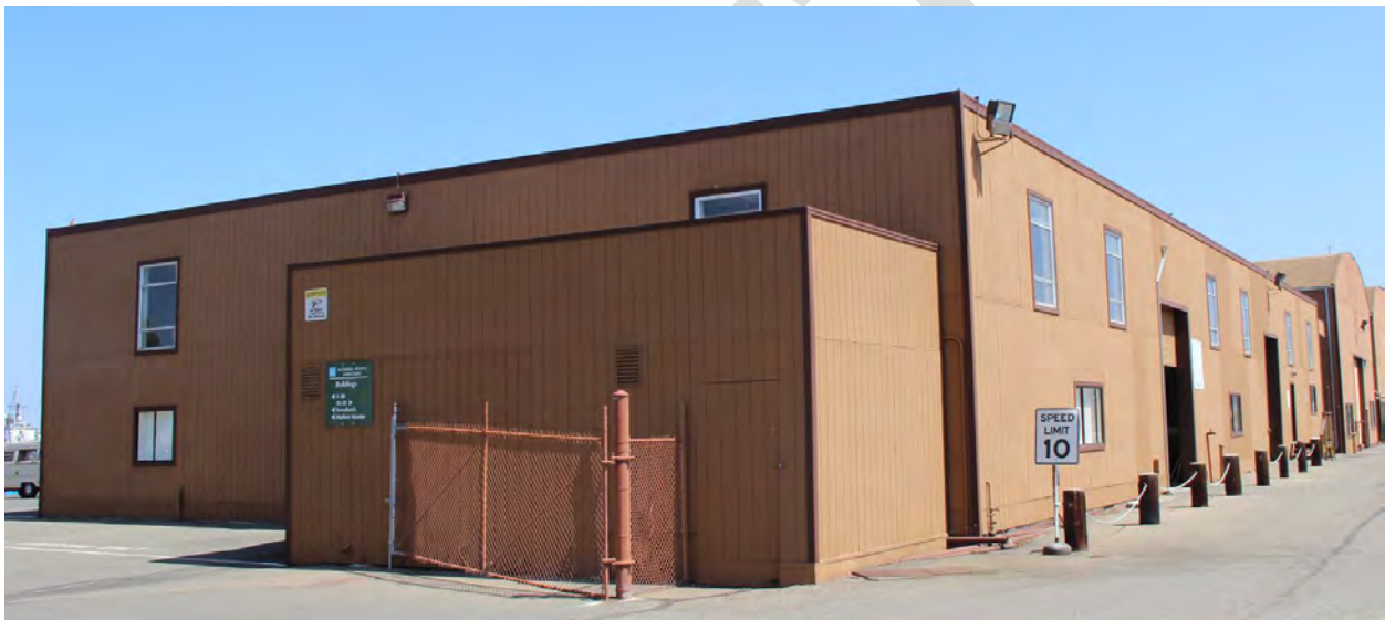
Figure 83. Building 32; south and east façades, view toward northwest, 2016.
