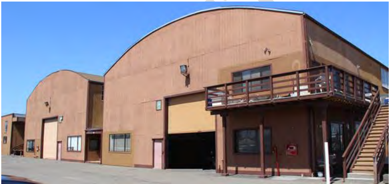
Figure 85. Buildings 33 (left) and 34 (right); view toward southwest, 2016.
