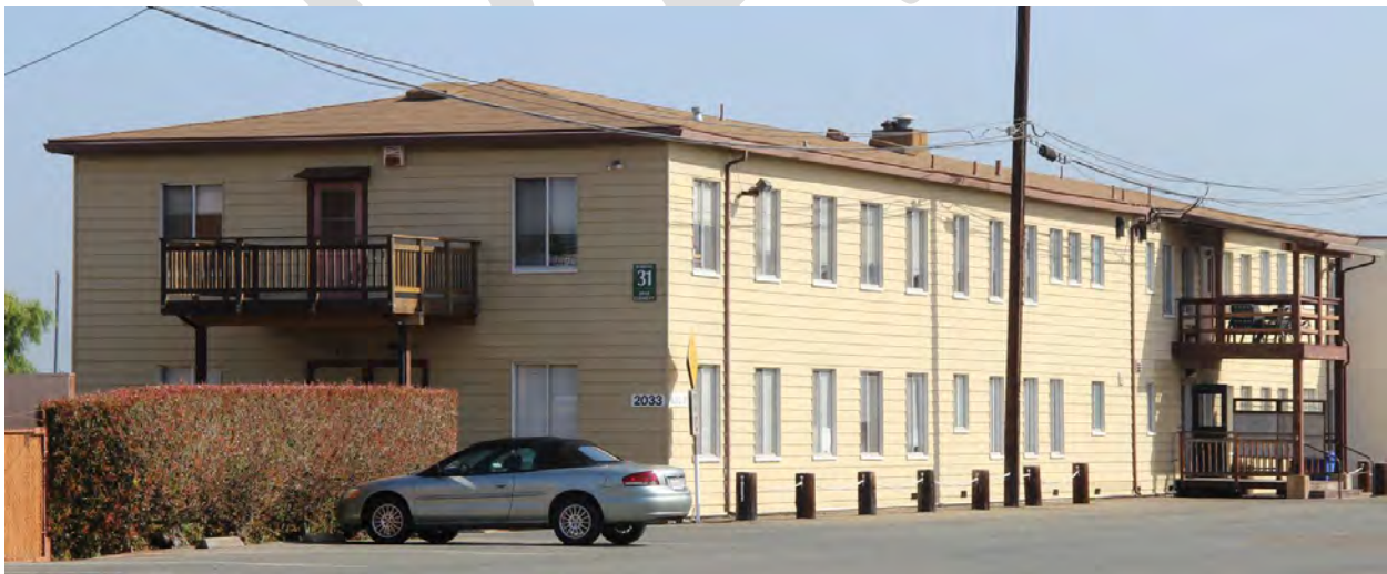
Figure 82. Building 31; south and east façades, view toward north, 2016.
