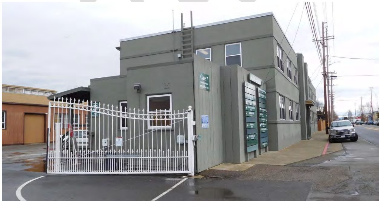
Figure 66. Building 21; south and west façades, view toward southeast, 2017.
