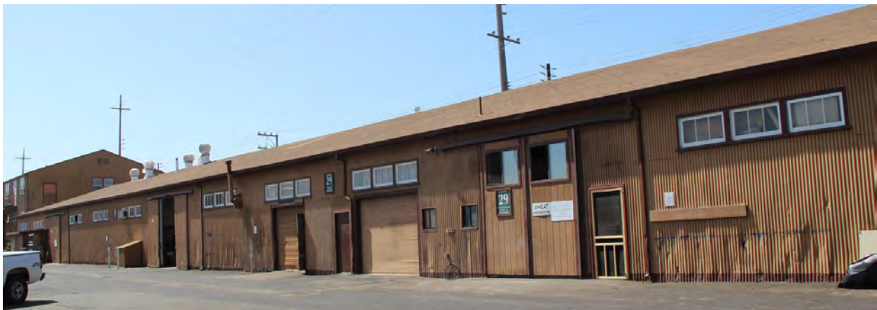
Figure 79. Building 29; north façade, view toward east, 2016.
