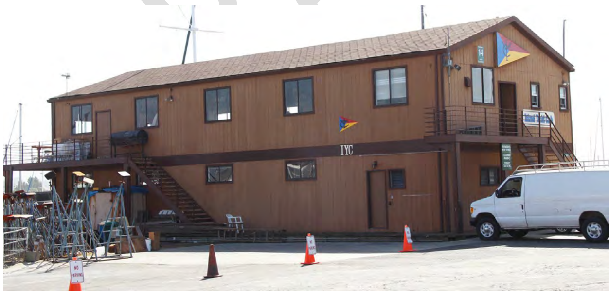
Figure 53. Building 14; south and west façades, view toward northeast, 2016.
