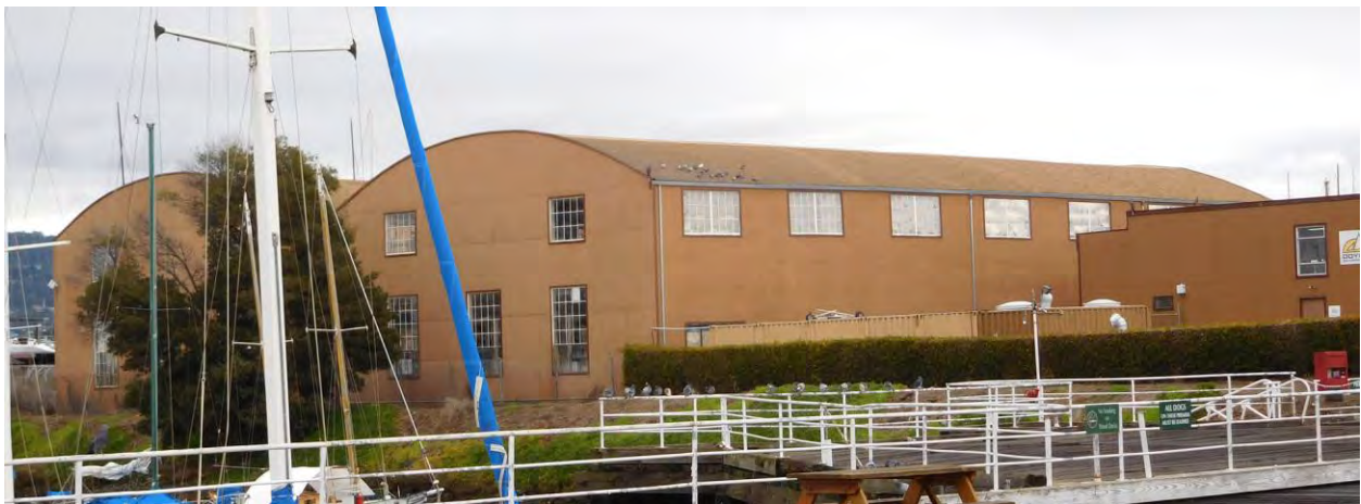
Figure 86. Buildings 33 (right) and 34 (left); view toward northeast, 2017.
