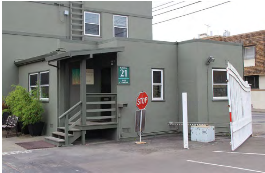
Figure 65. Building 21; north and west façades, view toward southeast, 2016.
