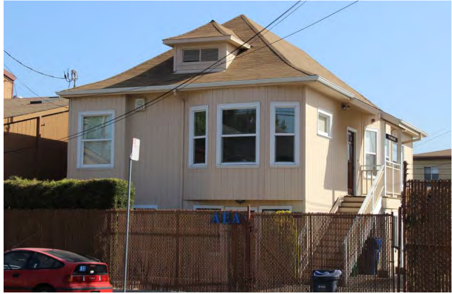
Figure 89. Building 37; south and east façades, view toward north, 2016.
