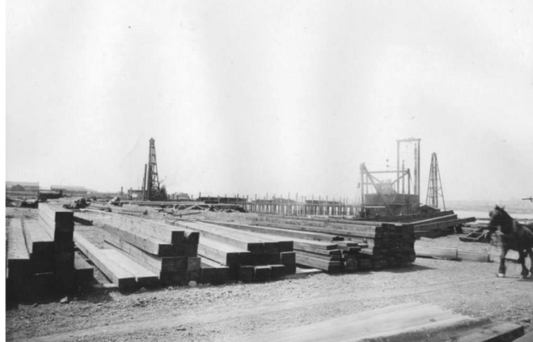
Figure 94. Barnes & Tibbitts shipyard under construction, 1917. Source: Oakland Public Library.
