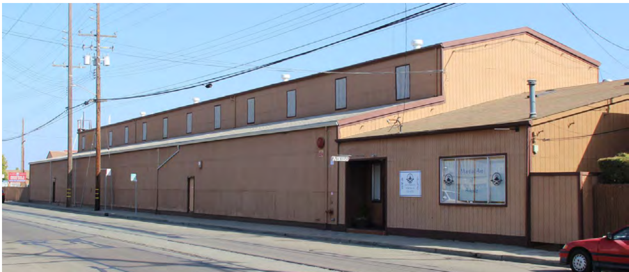
Figure 27. Building 1; south façade, view toward northwest, 2016.
