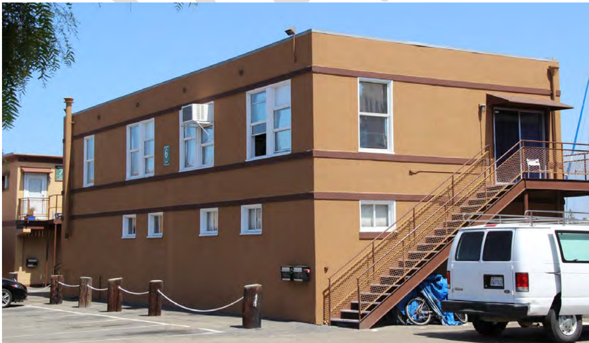
Figure 37. Building 6; south and east façades, view toward northwest, 2016.
