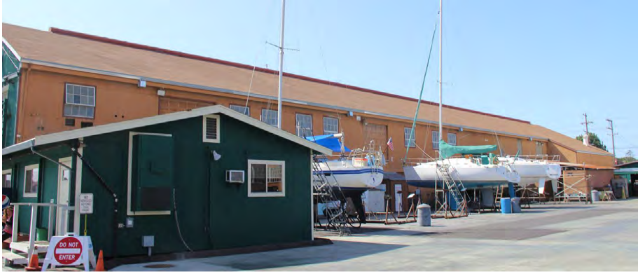
Figure 50. Building 12; west façade, view toward southeast, 2016. Note modular office building at left.
