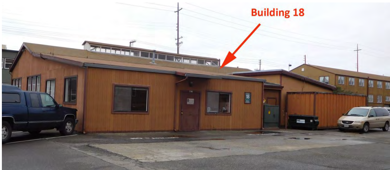
Figure 56. Building 18; north façade, view toward southwest, 2016
