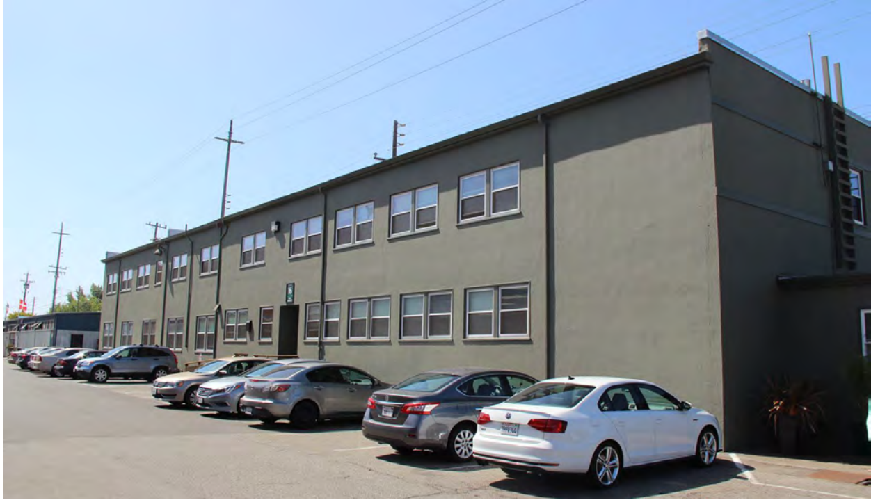
Figure 59. Building 16; north façade, view toward southeast, 2016.
