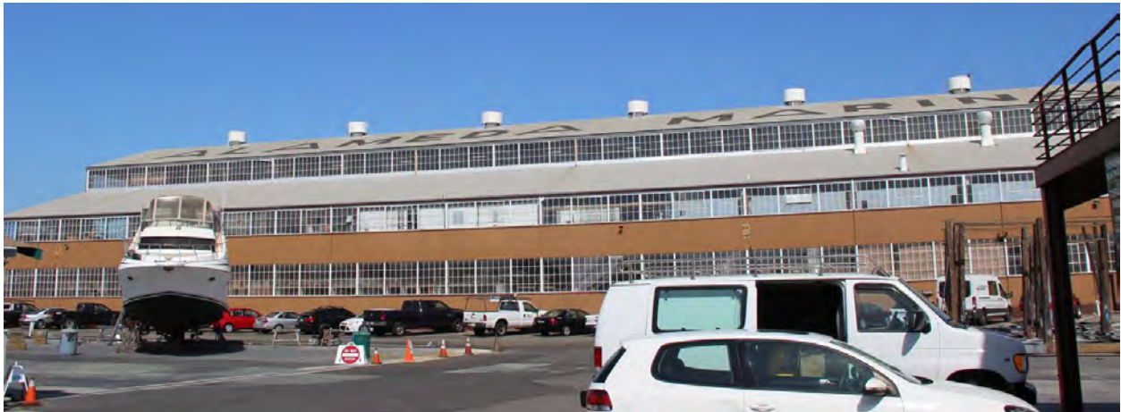
Figure 62. Building 19; view toward west, 2016
