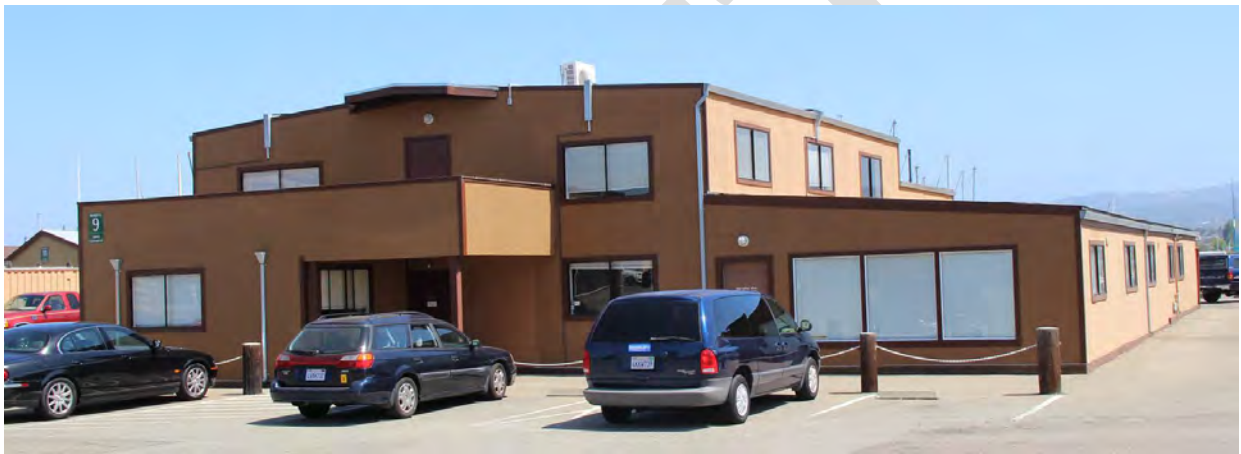
Figure 42. Building 9; south façade, view toward northwest.
