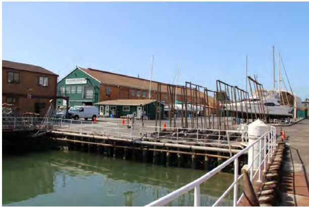
Figure 9. Typical bulkhead wharf at Alameda Marina, 2016.
