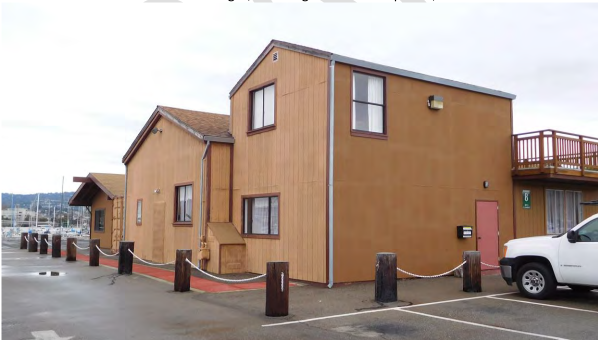
Figure 41. Building 8; south and west façades, view toward north, 2017.
