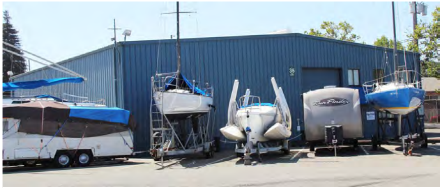
Figure 87. Building 35; view toward southeast, 2016.
