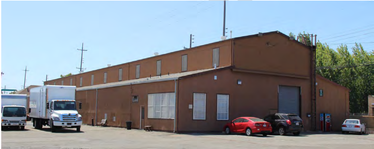
Figure 26. Building 1; north and west façades, view toward southeast, 2016.
