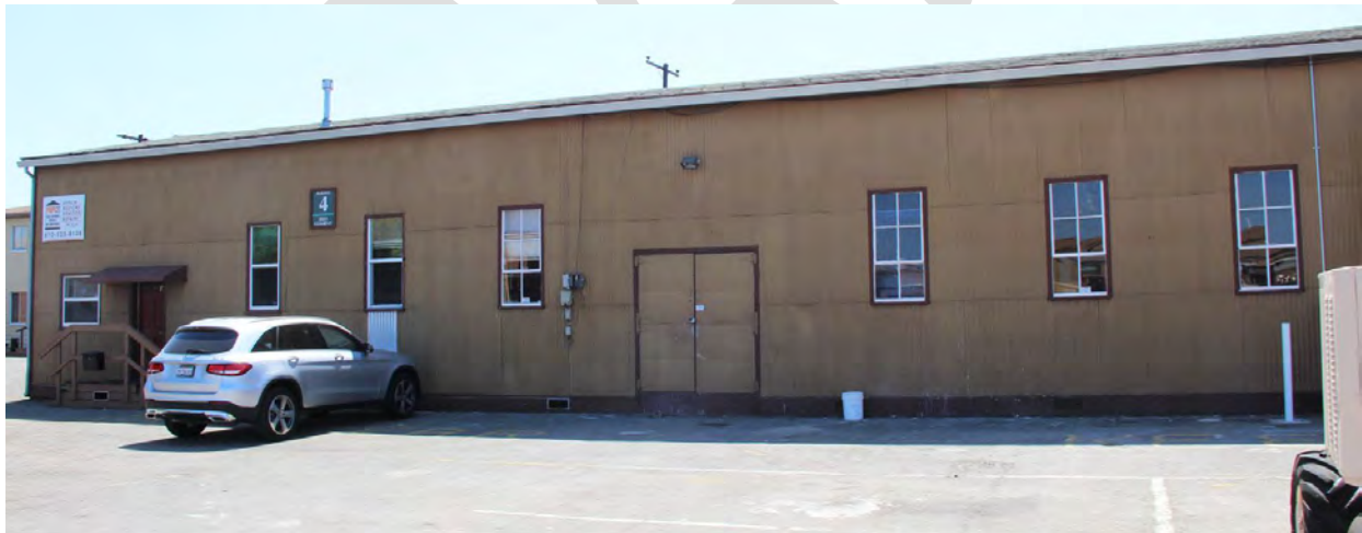
Figure 33. Building 4; west façade, view toward southeast, 2016.
