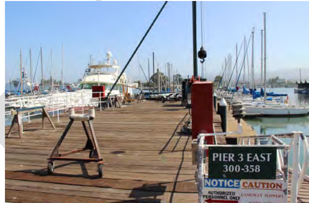
Figure 10. Typical pier at Alameda Marina, 2016.
