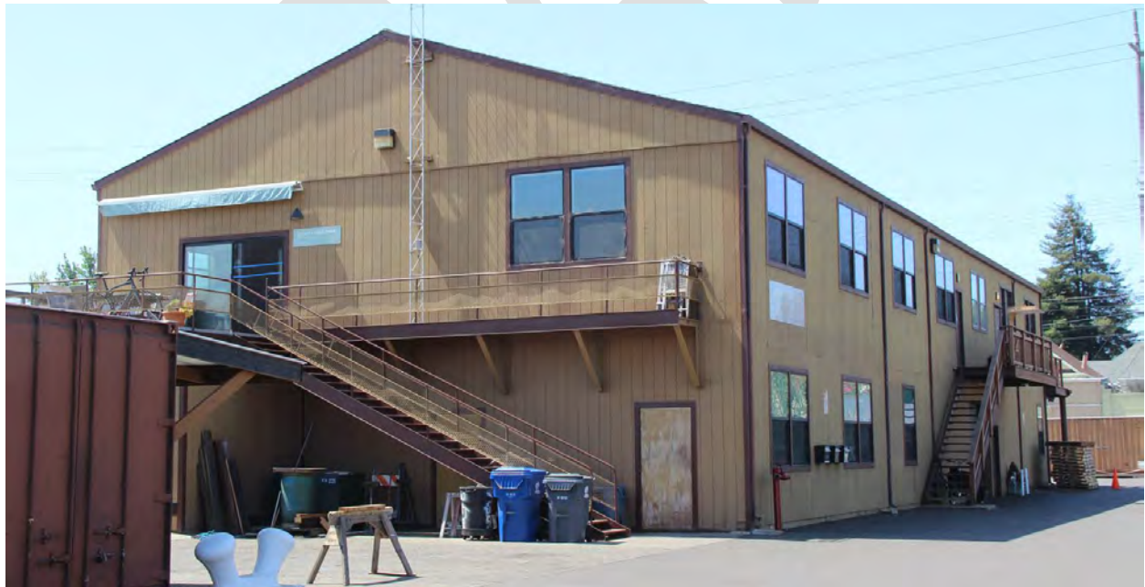
Figure 45. Building 10; north and west façades, view toward south, 2016.
