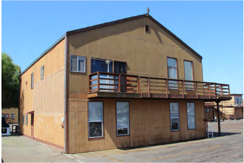
Figure 34. Building 5; north façade, view toward southwest, 2016.
