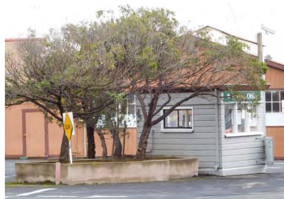
Figure 80. Building 30; view toward southeast, 2016.
