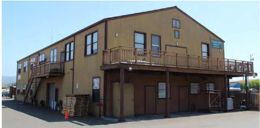
Figure 44. Building 10; south and west façades, view toward north, 2016.
