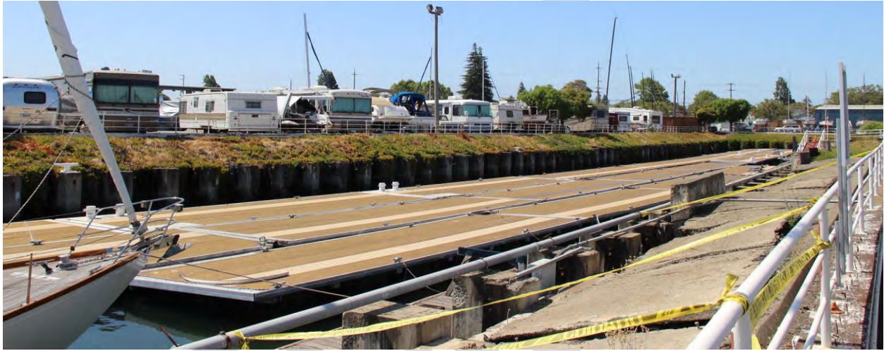
Figure 91. Graving dock; view toward southwest, 2016.
