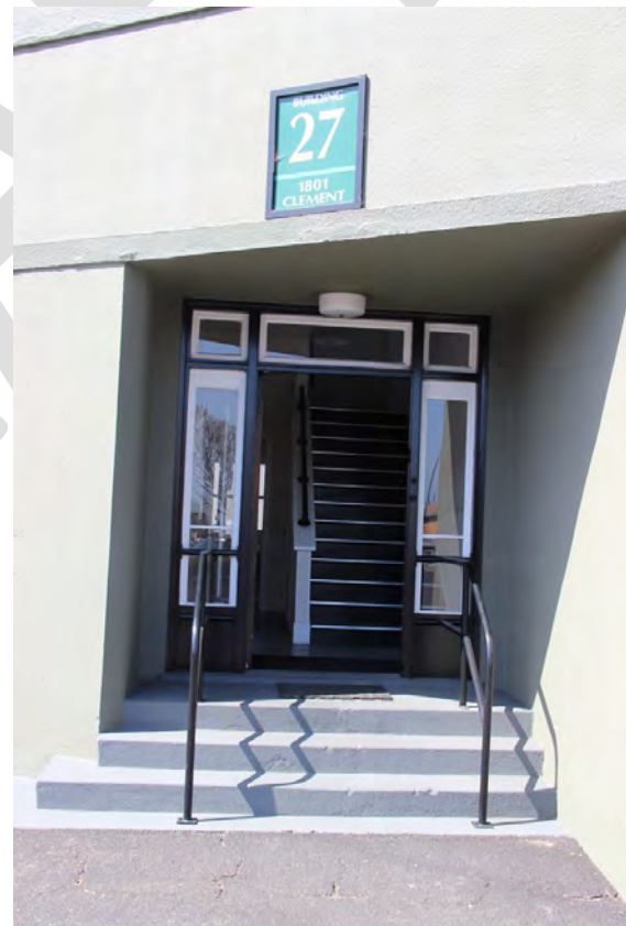
Figure 72. Building 27; main entrance, 2016.
