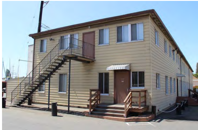
Figure 81. Building 31; north and west façades, view toward south, 2016.
