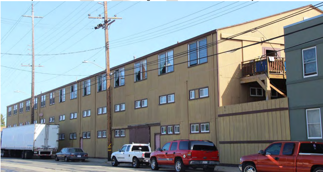
Figure 76. Building 28; south façade, view toward northwest, 2016.
