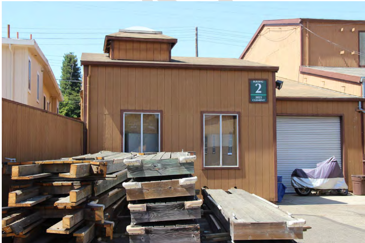
Figure 29. Building 2; north façade, view toward southeast, 2016.
