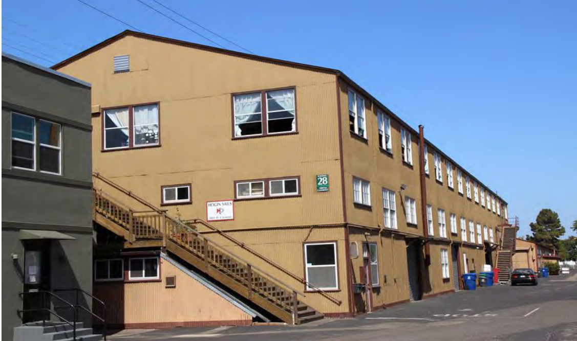
Figure77. Building 28; north and east façades, view toward west, 2016.
