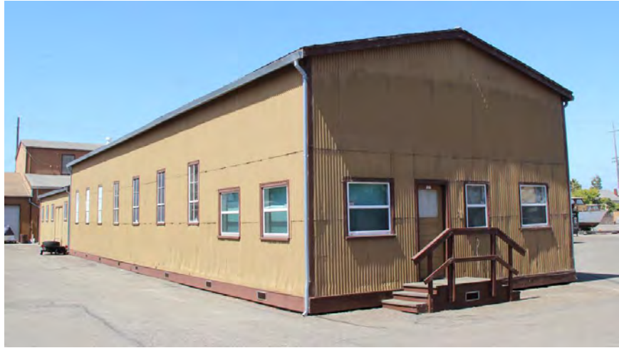
Figure 32. Building 4; north and east façades, view toward southwest, 2016.
