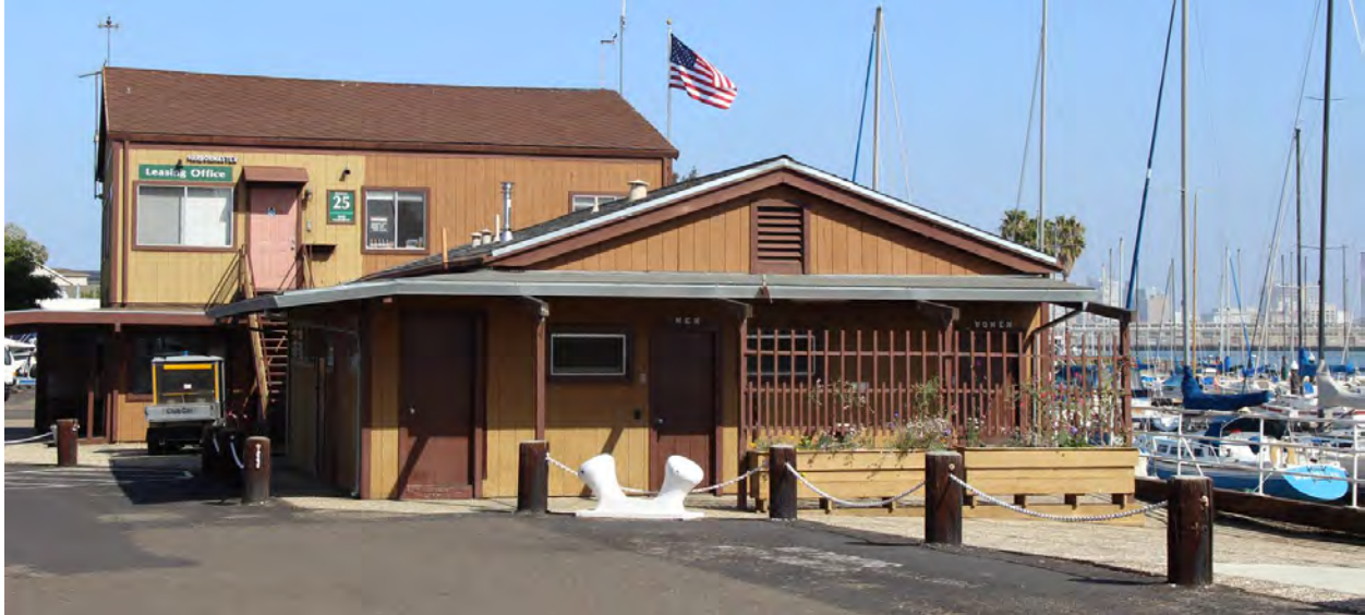
Figure 71. Buildings 25 (background) and 26 (foreground); view toward west, 2016.
