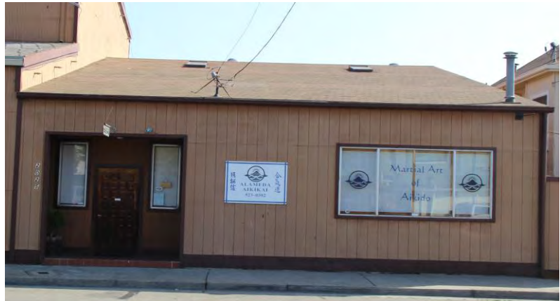
Figure 28. Building 2; south façade, view toward north from Clement Avenue. 2016.
