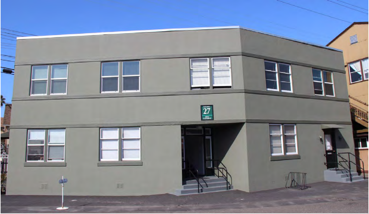
Figure 73. Building 27; north façade, view toward south, 2016.
