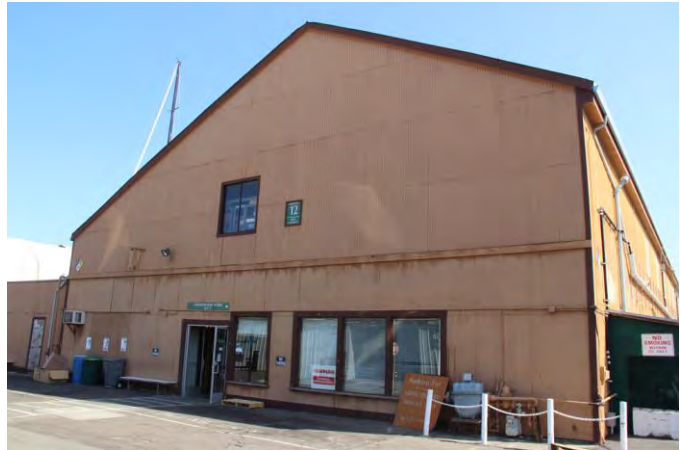
Figure 48. Building 12; south facade, view toward north, 2016.
