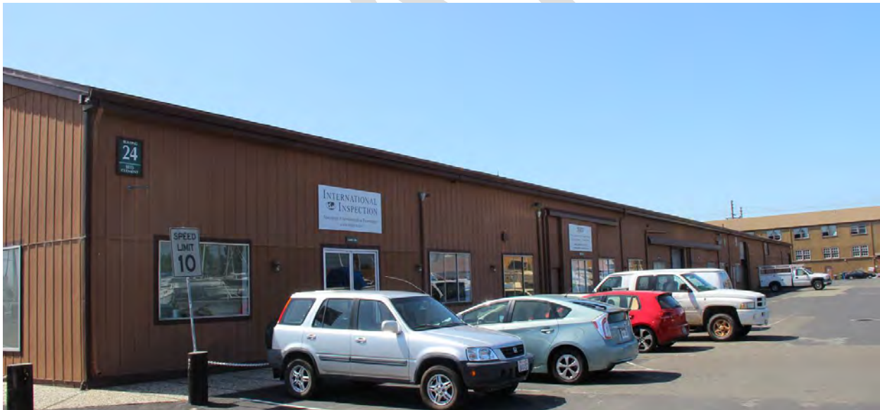
Figure 67. Building 24; west facade; view toward south, 2016.
