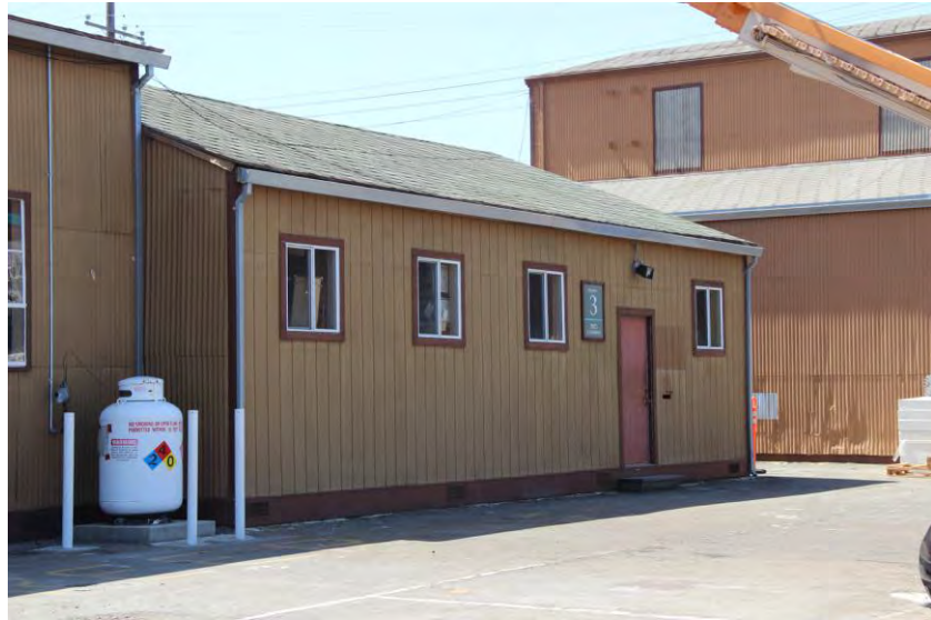
Figure 30. Building 3; west façade, view toward southeast, 2016.
