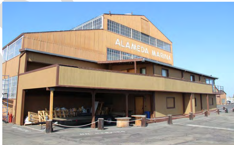
Figure 64. Building 20: view toward southwest. 2016.
