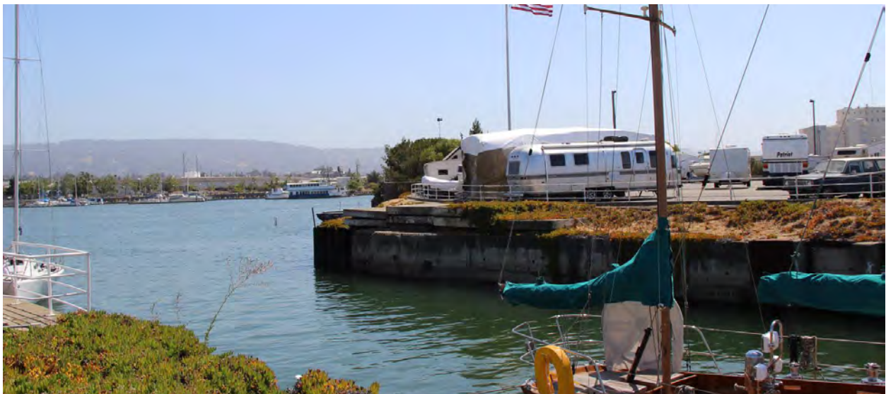
Figure 92. Graving dock; view toward northeast, 2016.
