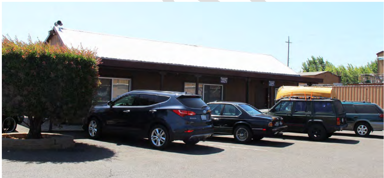
Figure 47. Building 11; west façade; view toward southeast, 2016.
