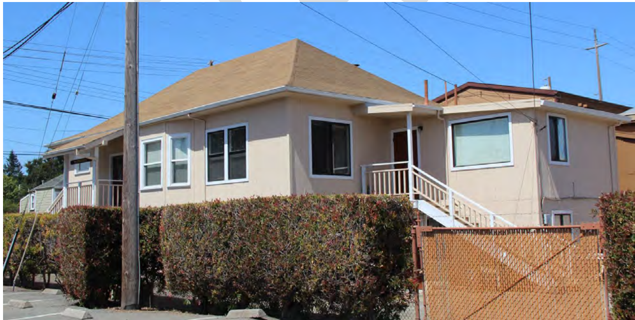
Figure 90. Building 37; north and east façades, view toward southwest, 2016.
