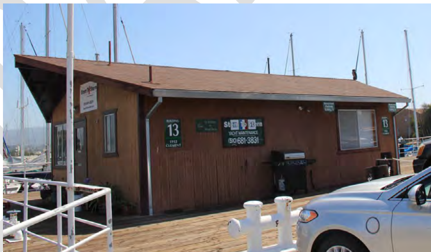
Figure 51. Building 13; south façade, view toward northeast, 2016.
