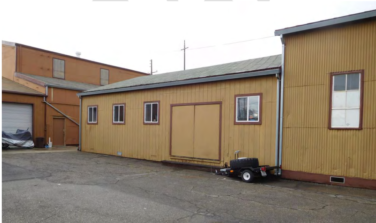
Figure 31. Building 3; east façade, view toward west, 2016.
