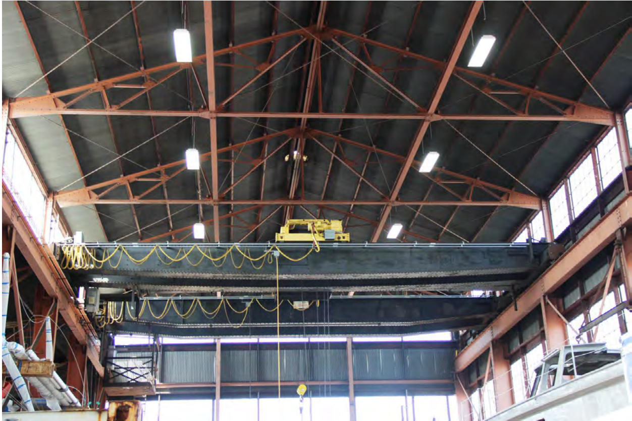
Figure 63. Building 19; view of interior trusses and gantry crane, 2016.
