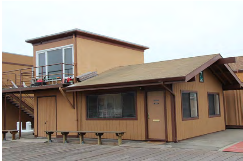
Figure 38. Building 7; north and west façades, view toward southeast, 2016.
