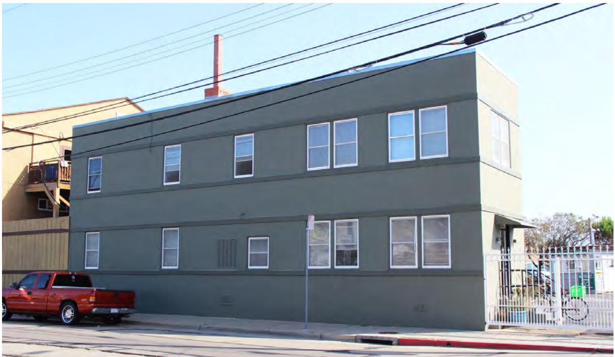
Figure 74. Building 27; south façade, view toward northwest, 2016.
