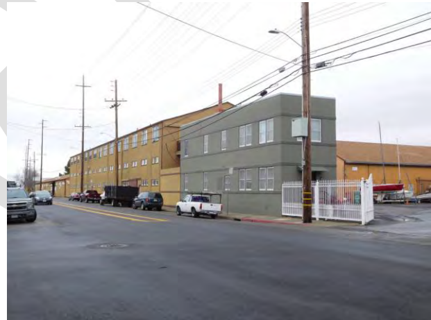
Figure 19. View westward along Clement Avenue showing Buildings 27, 28, and 29, 2017.
