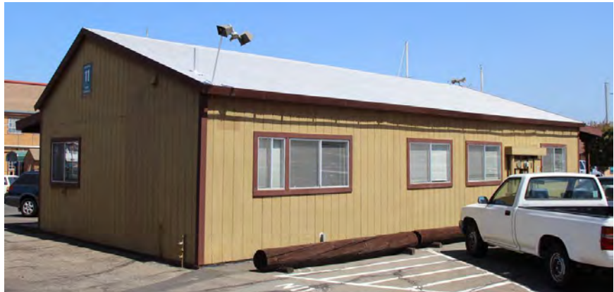
Figure 46. Building 11; south and east façades, view toward northwest, 2016.
