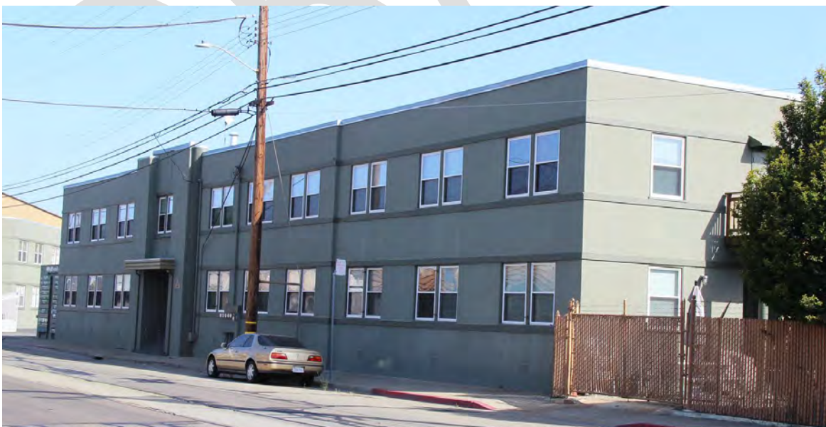
Figure 58. Building 16; south and east façades, view toward northwest, 2016.
