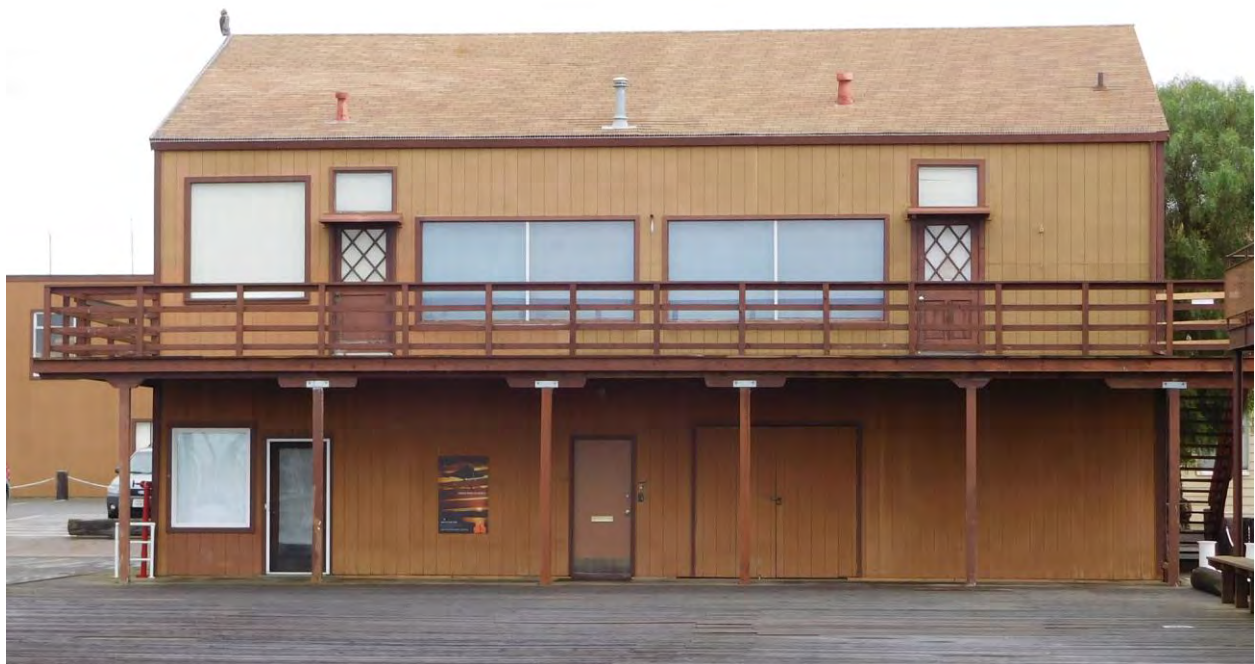
Figure 35. Building 5; west façade, view toward southeast, 2017.
