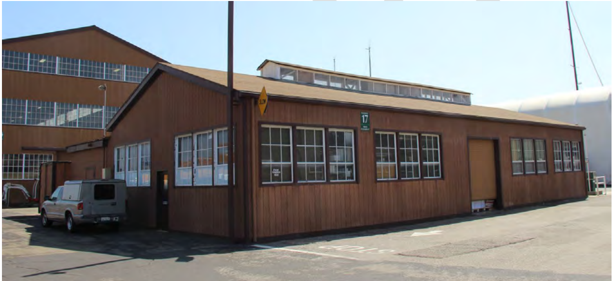
Figure 54. Building 17; south and west façades, view toward northeast, 2016.
