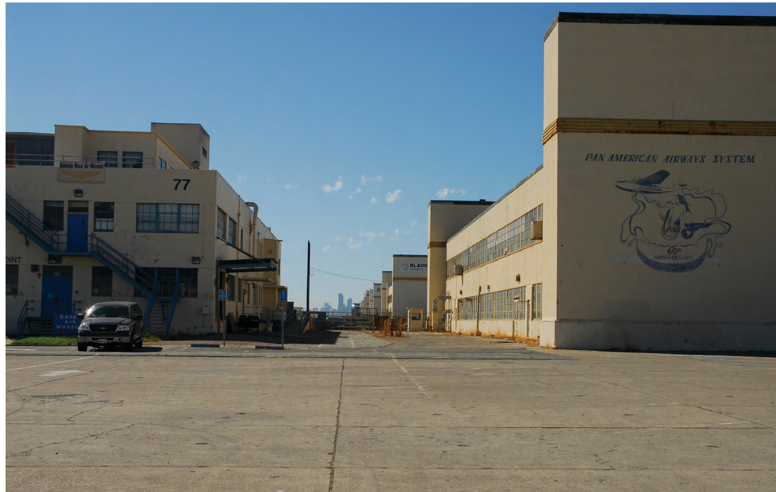
EXISTING BUILDING 77 (LEFT) AND 41 (RIGHT)
