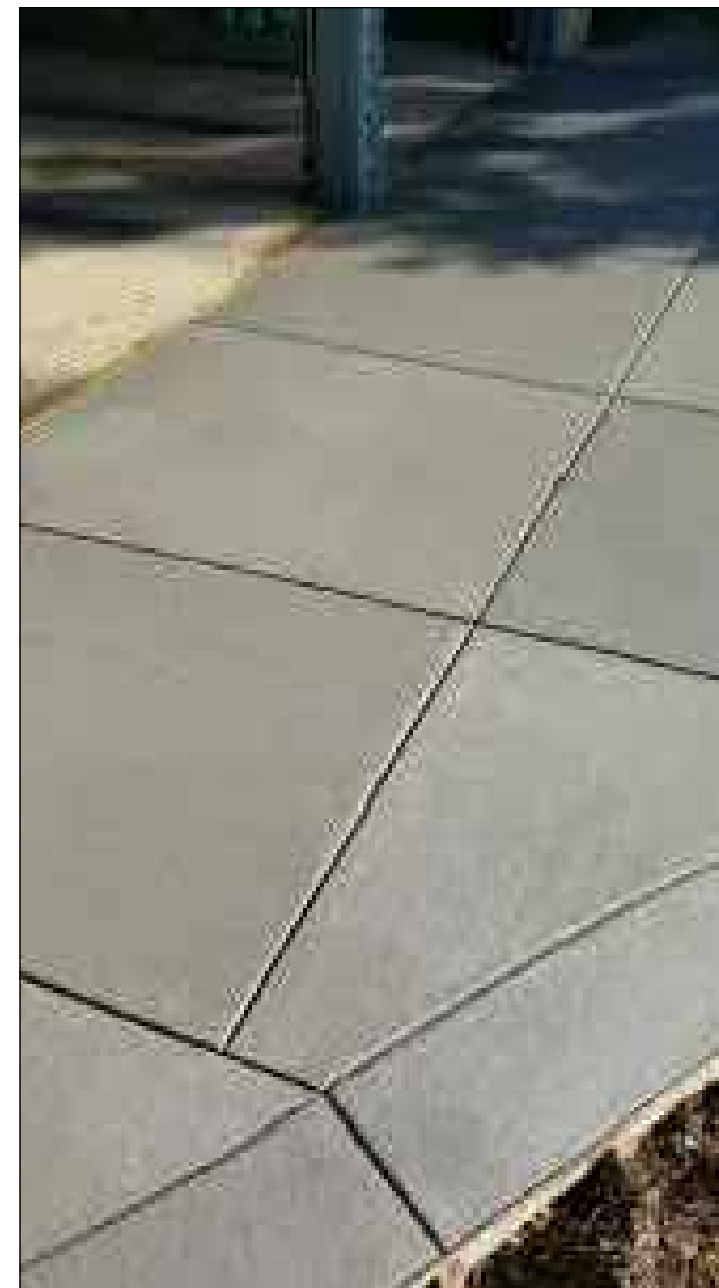
CONCRETE PAVING WITH MEDIUM BROOM FINISH AND DEEP CONTROL JOINT SCORING
