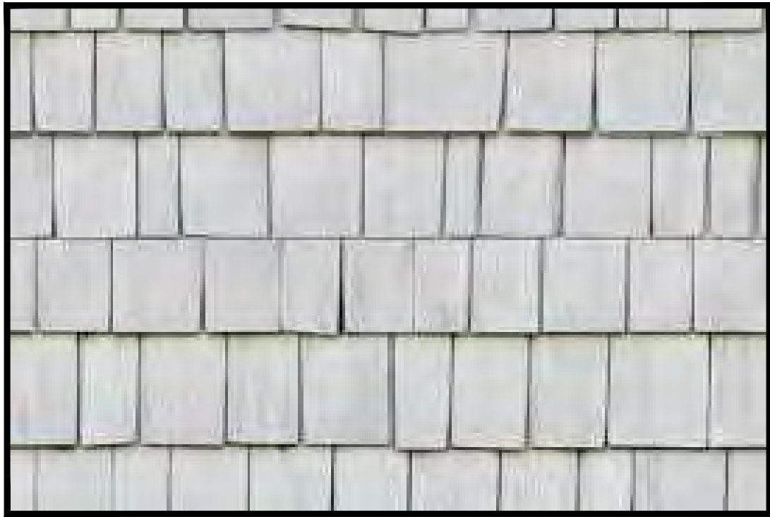
SIDING 2 SHINGLE CEMENT BOARD SIDING PAINT: KELLY MOORE COLOR: SAN FRANCISCO FOG (KM5822)
