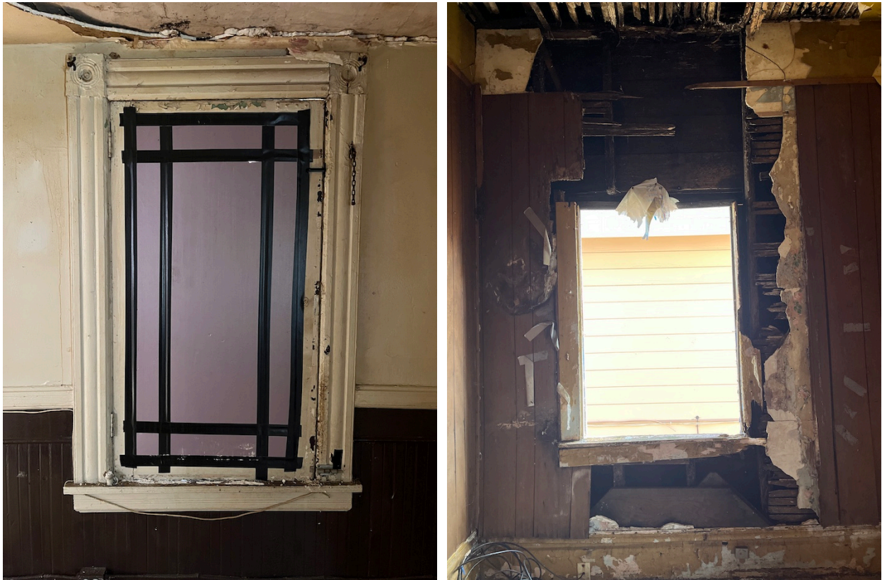
Figure 13. (Left) View of 1st floor window from the East wall interior. Note window is racked and boarded up from the interior due to missing panes (GA, June 2025); (Right) View of 2nd floor window from the North wall interior. Note missing window and framing damage (GA, June 2025).
