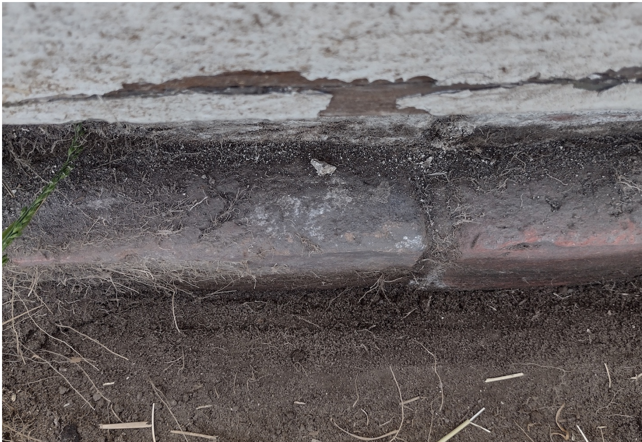
Figure 7. View of the brick foundation at the front (East) facade of 1711 Arbor Street (GA, June 2025)
