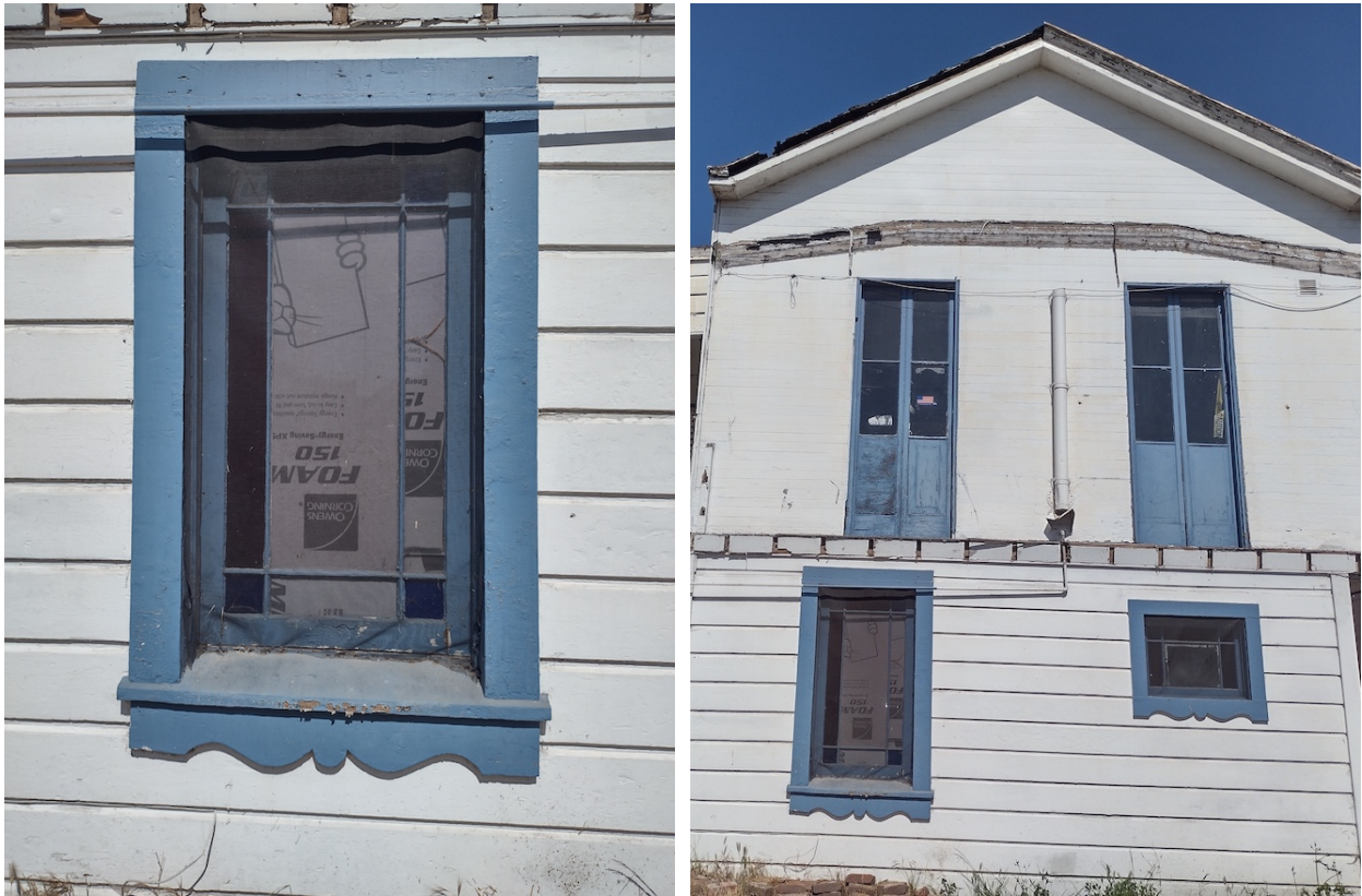
Figure 9. (Left) View of 1st floor window at East elevation. Note window is boarded up from the interior due to missing panes (GA, June 2025); (Right) View of window windows and doors on the East elevation (GA, June 2025).
