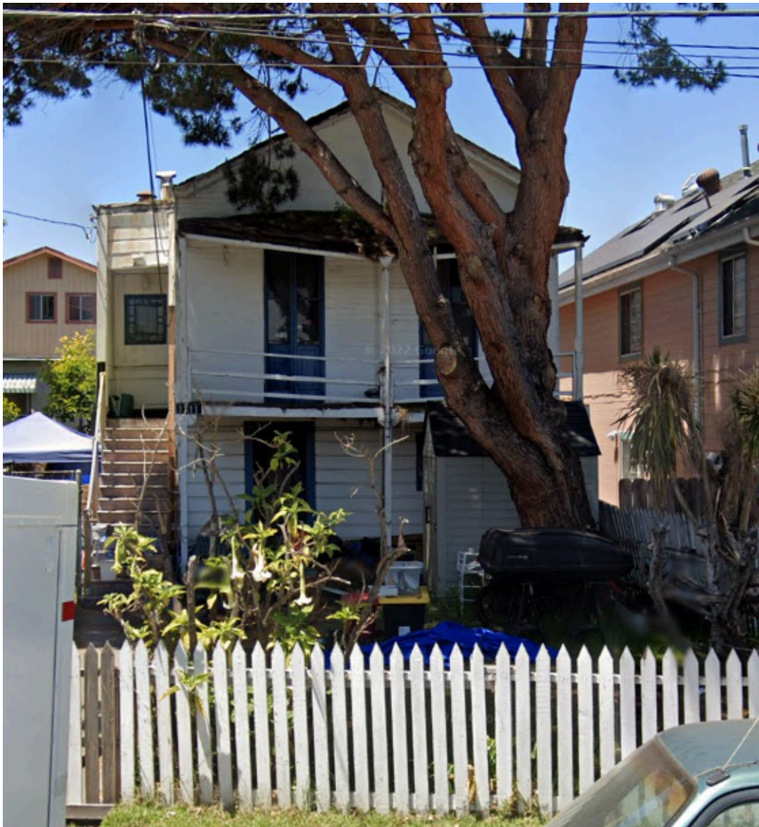
Figure 6. Front porch in 2022; note that the tree is leaning onto the porch, compromising its structural integrity (Google Maps)
