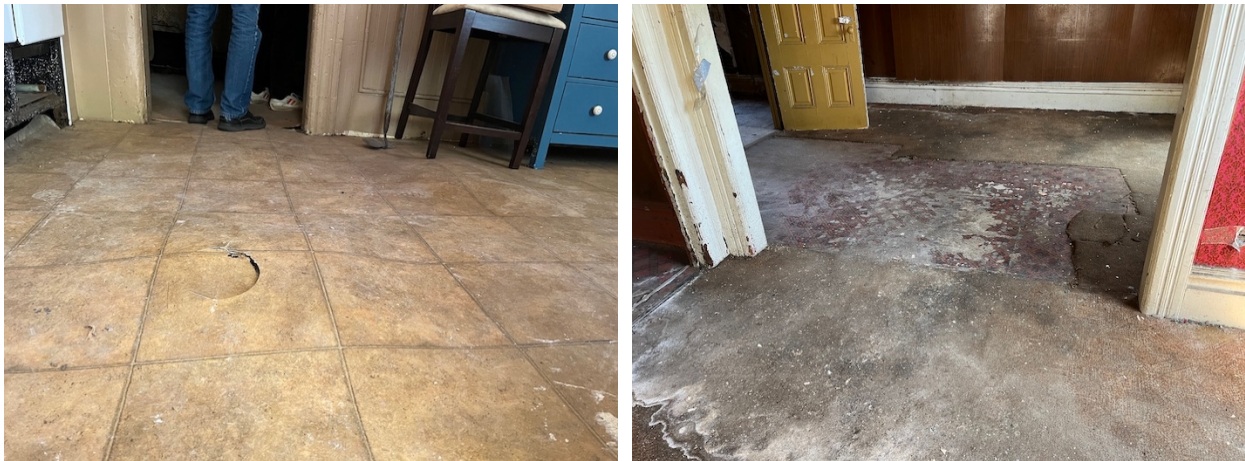
Figure 11. (Left) View of bubbling and warped linoleum at 1st floor kitchen (GA, June 2025); (Right) View of stained and deteriorated carpeting and linoleum at 2nd floor reception hall and living room (GA, June 2025).
