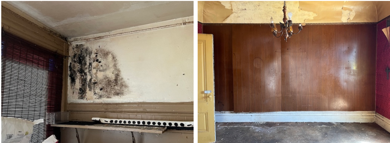
Figure 12. (Left) View of mold on West wall of 1st floor kitchen (GA, June 2025); (Right) View of warped wood paneling at North wall of 2nd floor living room (GA, June 2025).
