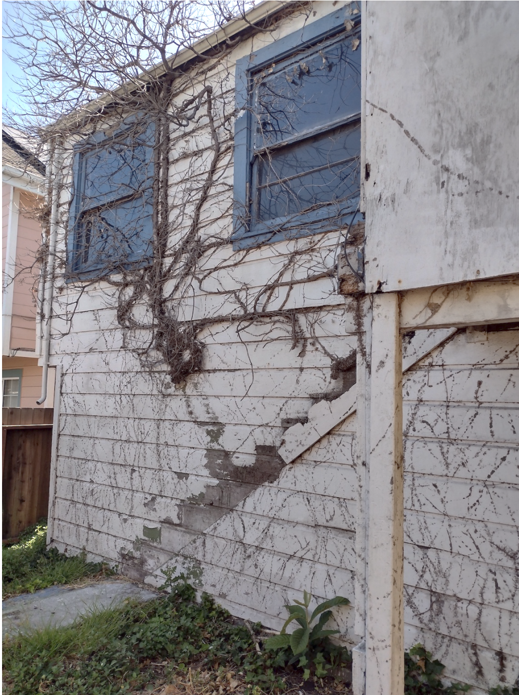
Figure 8. View of vine damage at the rear (West) facade of 1711 Arbor Street (GA, June 2025)
