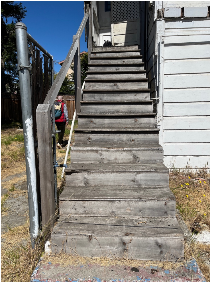
Figure 10. View of exterior staircase at East elevation. Note deteriorated and cracked wood (GA, June 2025)
