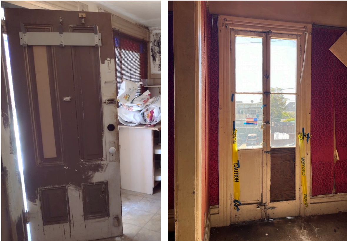
Figure 14. (Left) View of 1st floor entrance door from the South wall interior. Note failing paint and weathered wood elements (GA, June 2025); (Right) View of 2nd floor door from the East wall interior. Note deteriorated wood elements, failing paint, and plywood at the lower panel of the South-side door (GA, June 2025).
