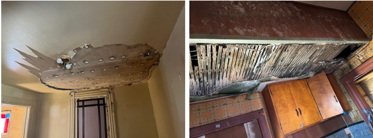
Figure 15. (Left) View of failed plaster at ceiling of 1st floor living room (GA, June 2025); (Right) View of failed plaster and deteriorated wood lath at ceiling of 2nd floor kitchen (GA, June 2025).
