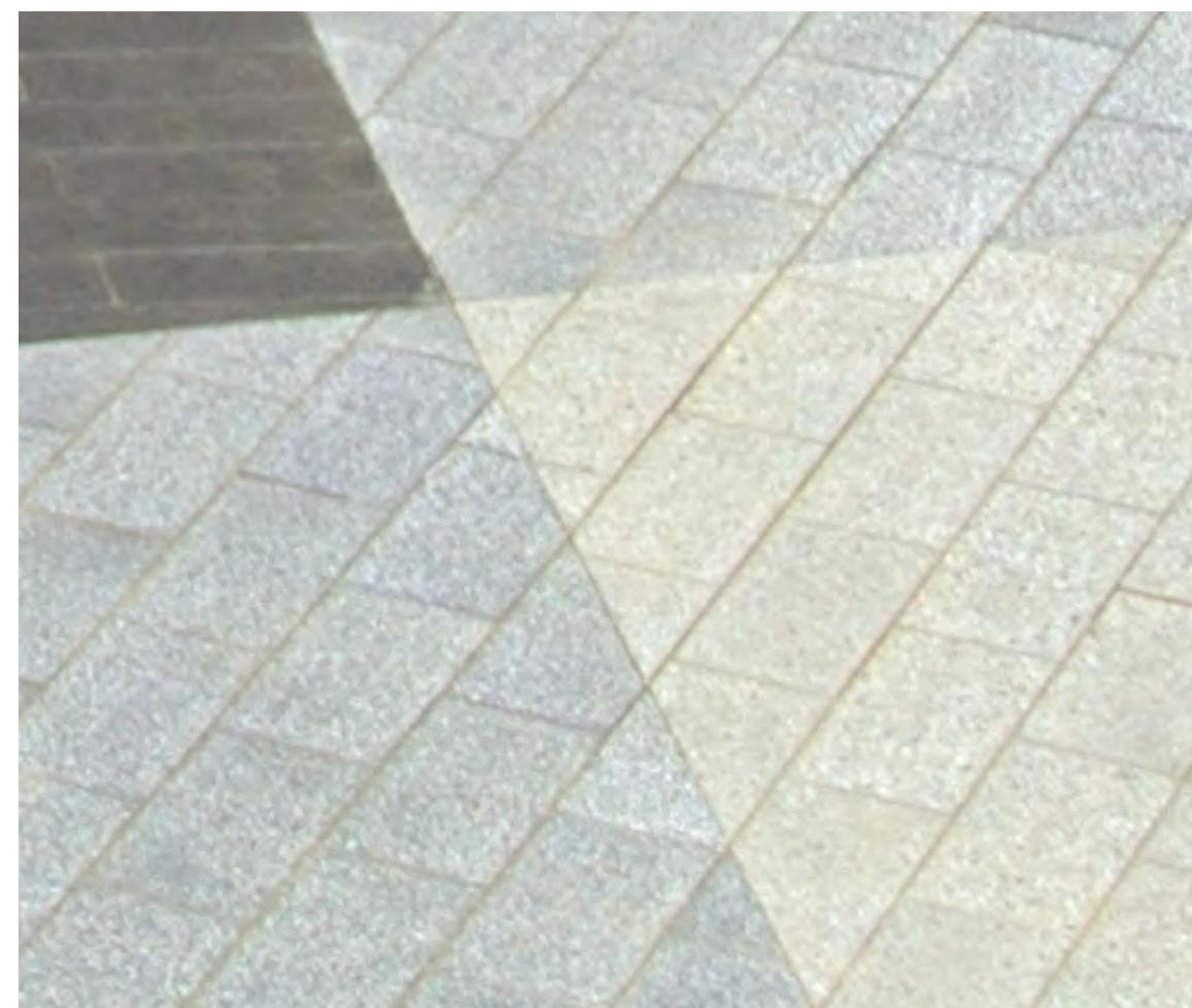
Basalite 4x8 Permeable Pavers, open joints UNIT PAVERS
