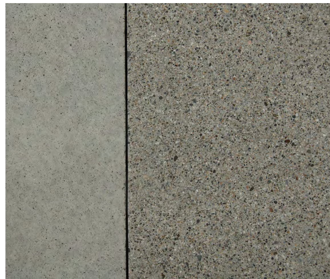
Light sandblast finish, integral color, saw-cut joints CONCRETE
