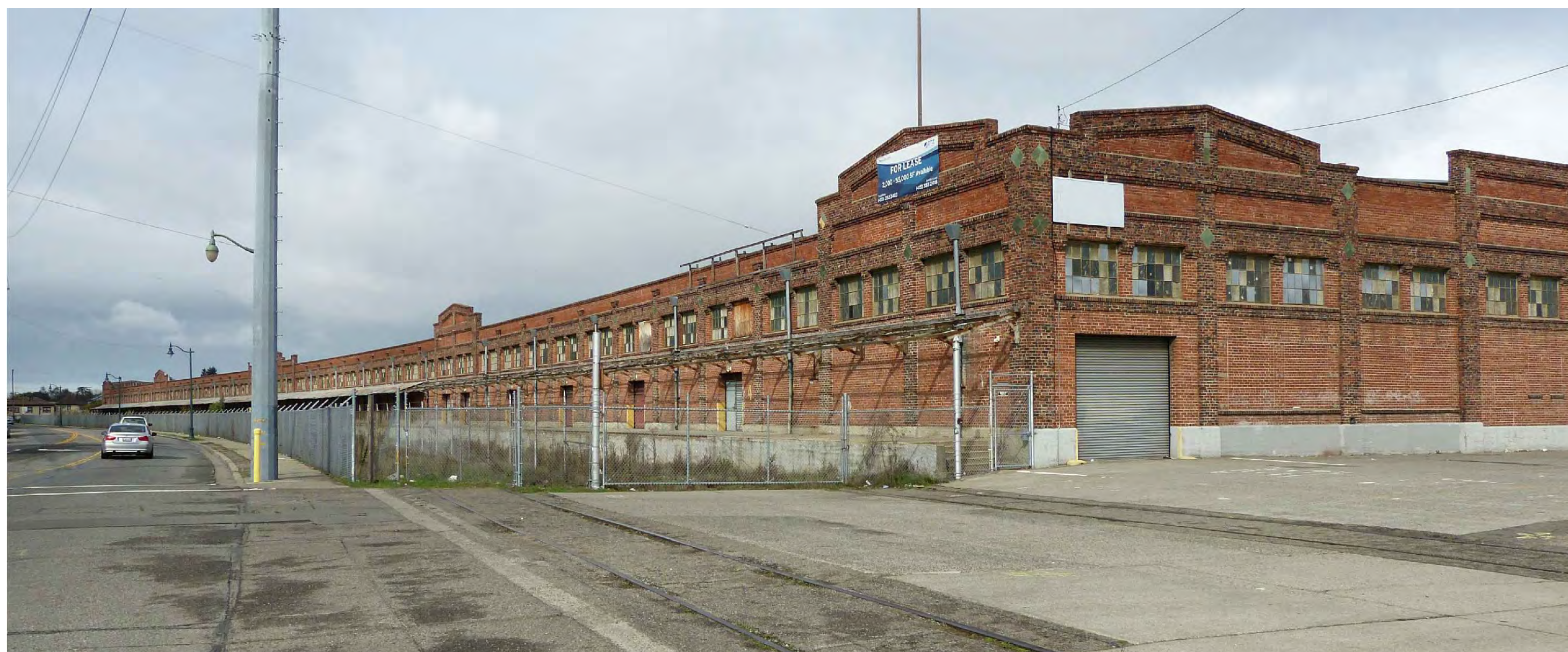
VIEW 3 - EXISTING CONDITION VIEW FROM BUENA VISTA AVE AND ENTRANCE RD
