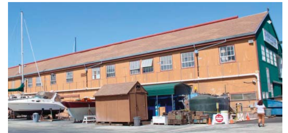
View of Building 12, East Facade
