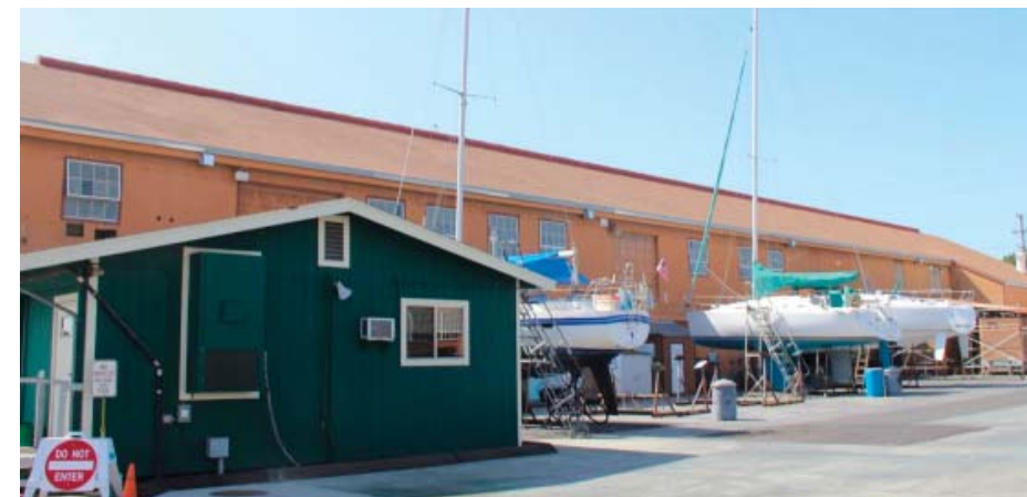
View of Building 12, West Facade
