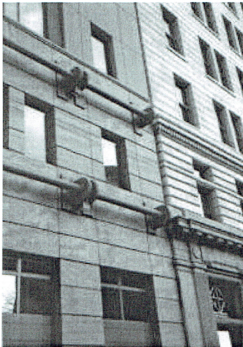
Guideline 4.2: Encouraged - Continue the horizontal lines and vertical rhythm of existing neighboring buildings.
