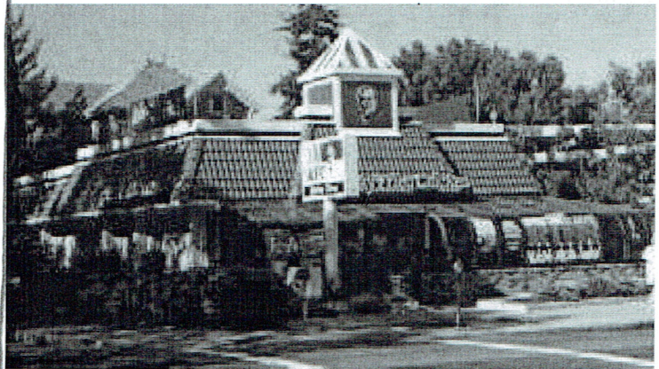
Guideline 4.4: Discouraged - Do not design buildings or storefronts in “corporate” or “franchise” styles.
