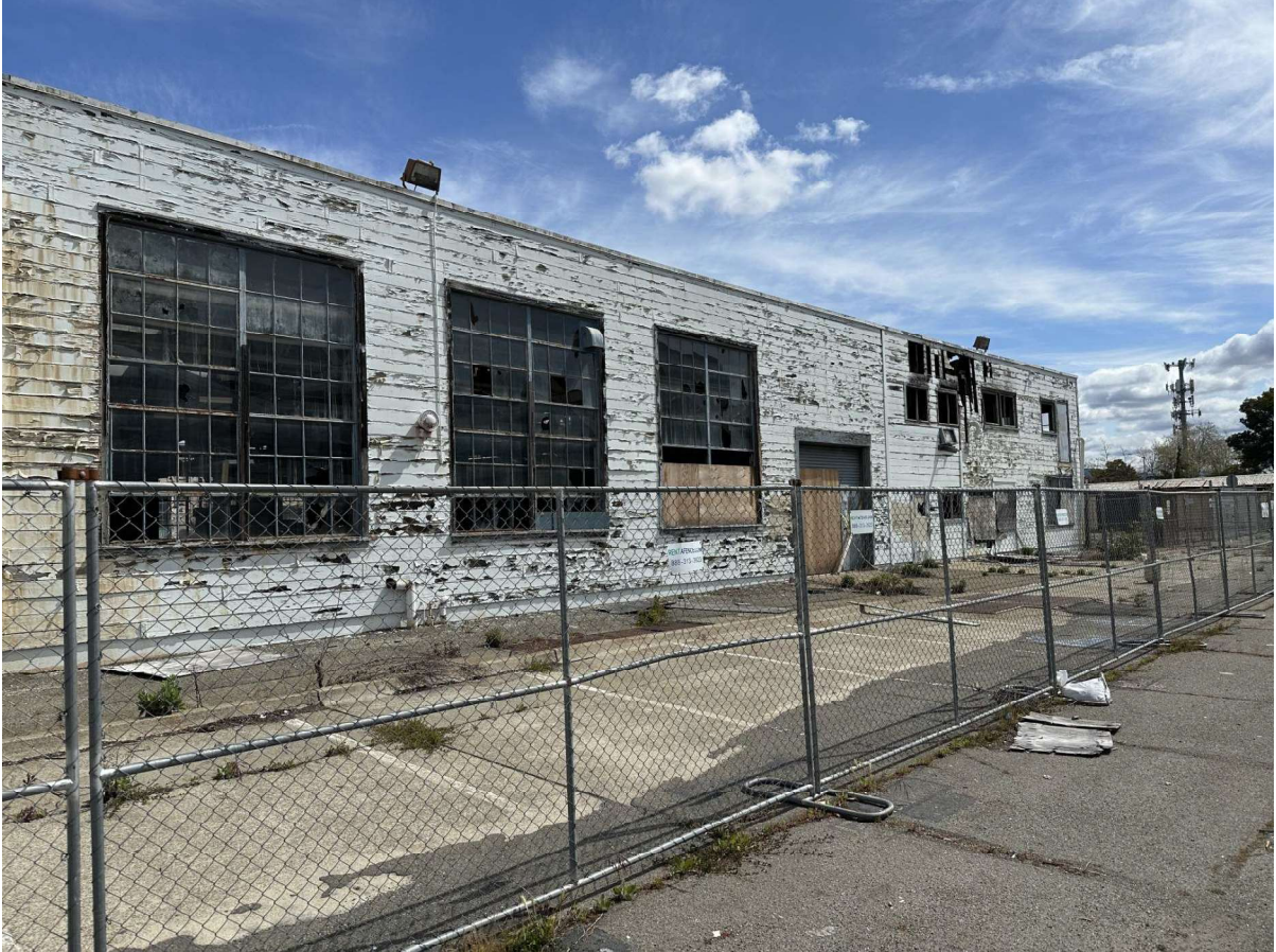
Figure A.9 - Exterior Siding and Windows.
