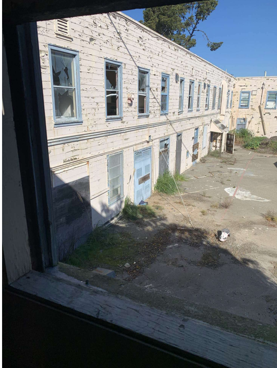
Figure A.8 - Exterior siding and windows.
