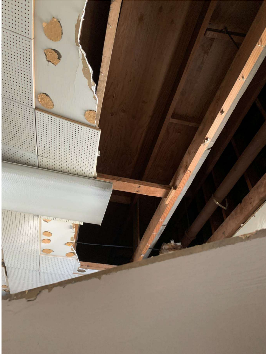
Figure A.1 - Exposed roof framing and sheathing.
