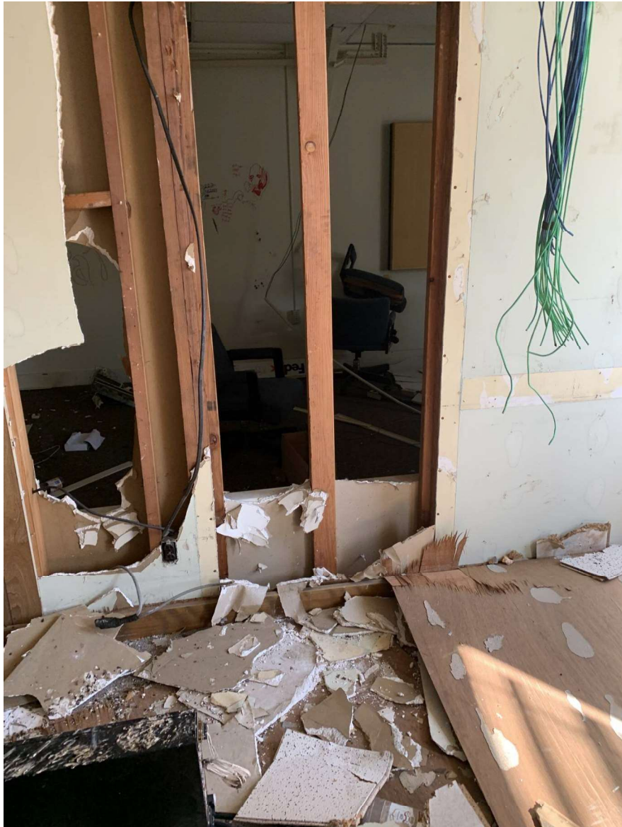
Figure A.2 - Exposed wall studs.
