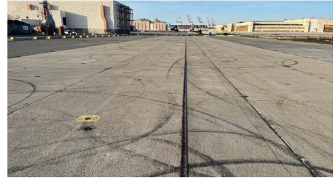
Existing Concrete Paving
