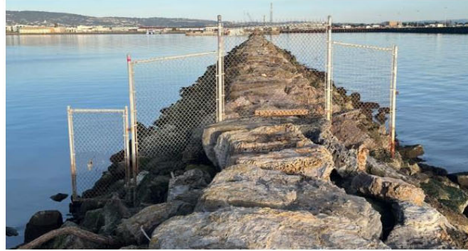
Stone Jetty at the South End of Site
