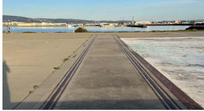
Rails Embedded in Concrete
