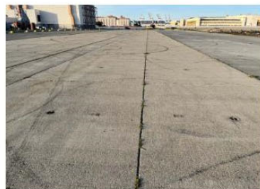
Existing Concrete Re-Use
