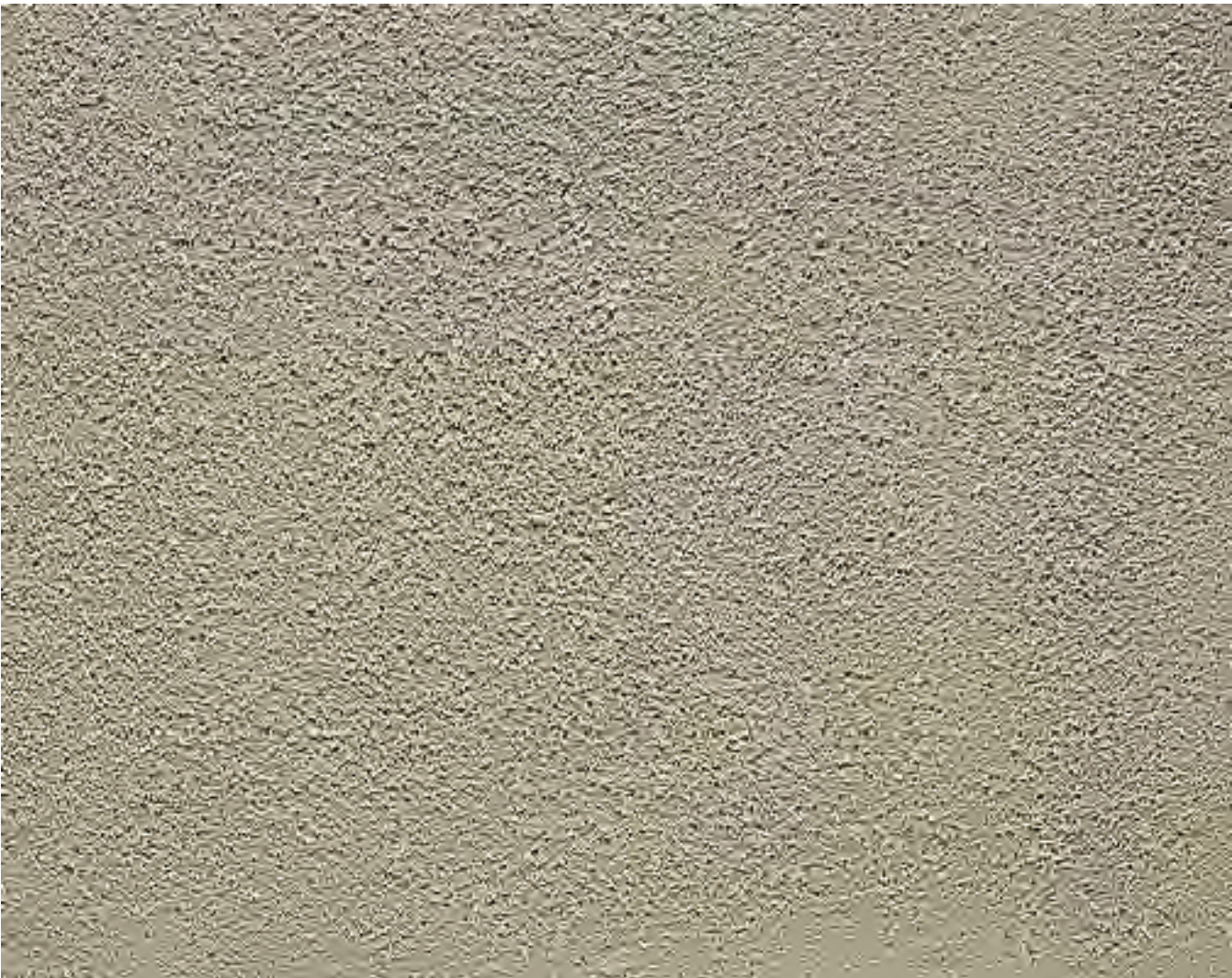
SAND FINISH STUCCO (SEE ELEVATIONS FOR COLORS)
