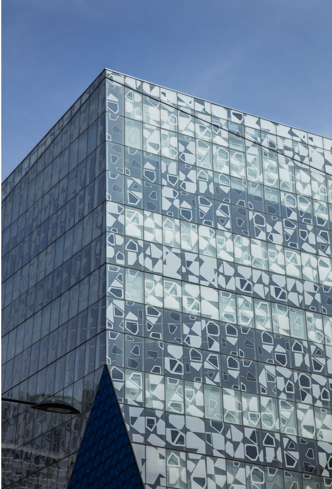
The patterns etched on windows of a Ryerson University building in Toronto were employed for aesthetic reasons, but act as collision deterrents. Photo: Richard Barnes
