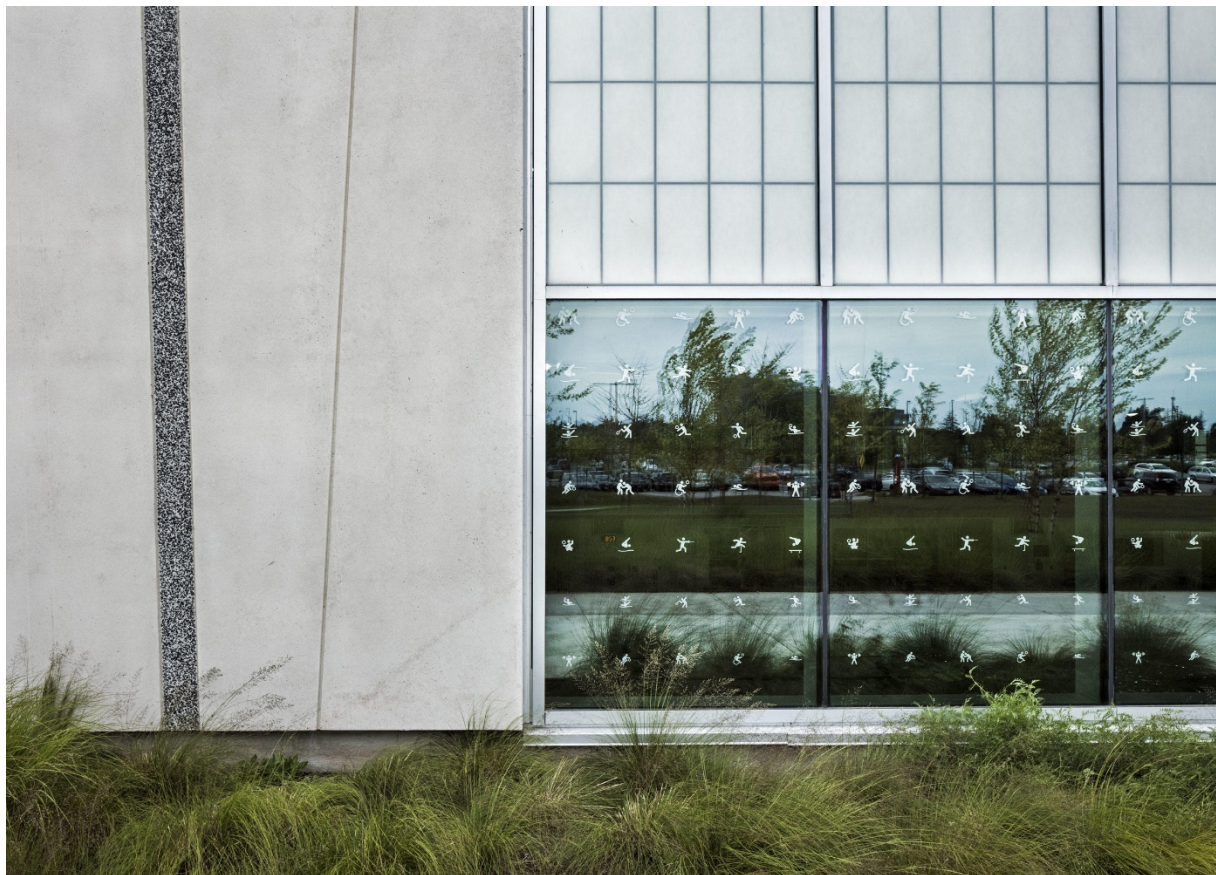
The Toronto Pan Am Sports Centre building in the suburbs of Toronto was designed with bird-strike mitigation in mind. Whimsical etchings of athletes appear on every panel of exterior glass. Photo: Richard Barnes
