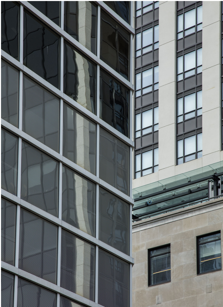
The etchings on the windows of this building in downtown Toronto resemble Venetian blinds and make the reflective surface visible to birds. Photo: Richard Barnes
