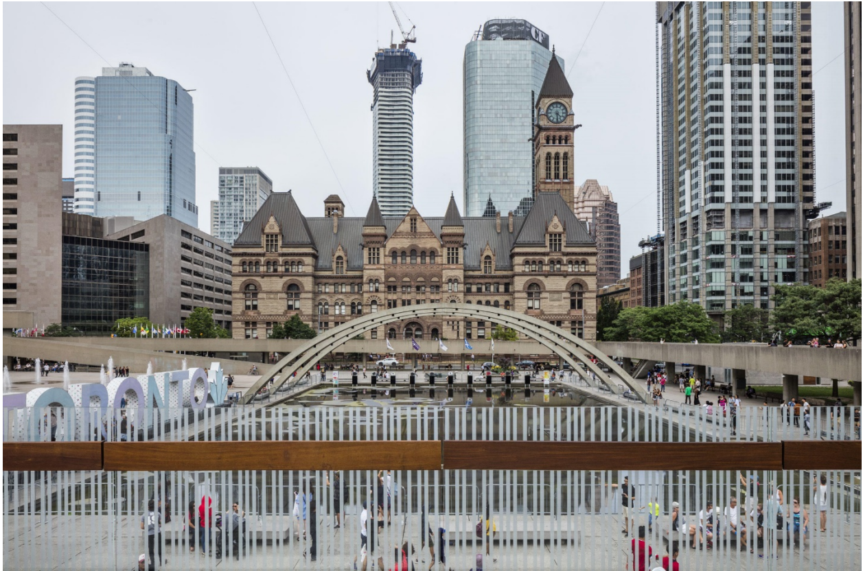
The fritted glass panels at a skate pavilion across from the old city hall were intentionally installed to alert birds to the boundary. Photo: Richard Barnes
