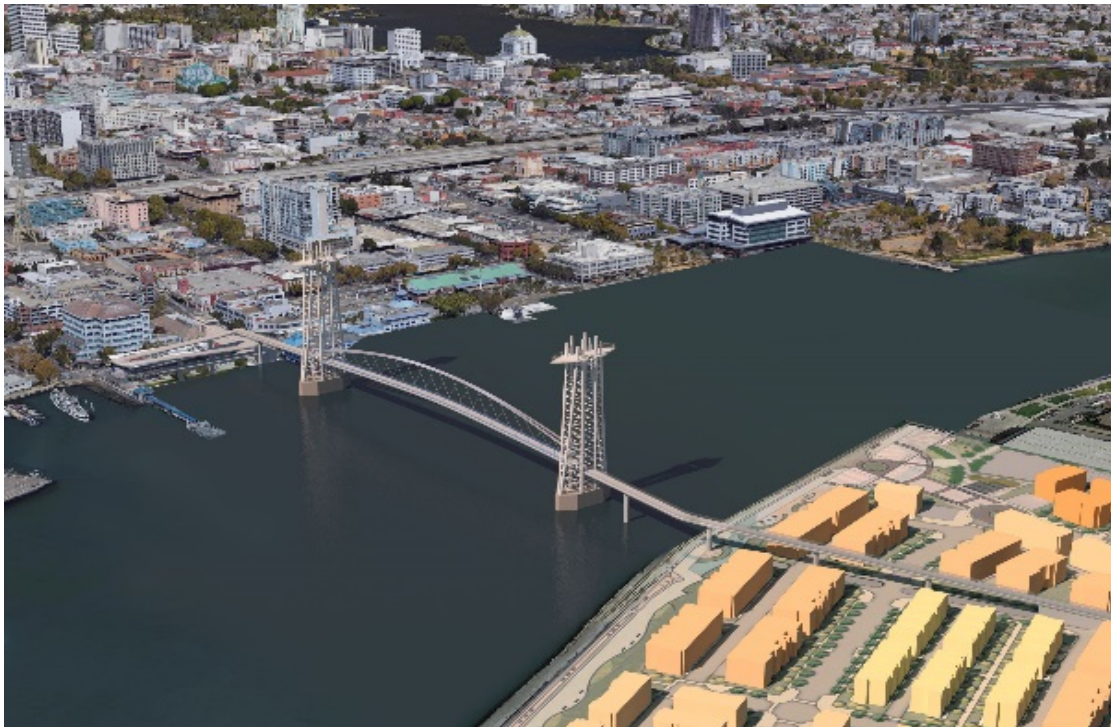
The bridge graphic shown above illustrates a concept for a bicycle and pedestrian lift bridge connecting Alameda Landing and Jack London Square and a future A's Stadium. The lift bridge allows the bridge to be raised to allow the Coast Guard cutters to access Coast Guard Island and the San Francisco Bay.
