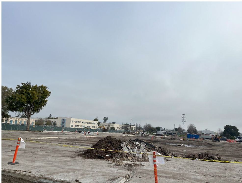
Photos taken at 11:00 AM Monday, January 6, 2025, looking east from Saratoga Street.
