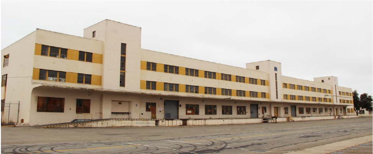
Figure 10. North façade of Building 8; view toward southwest.
