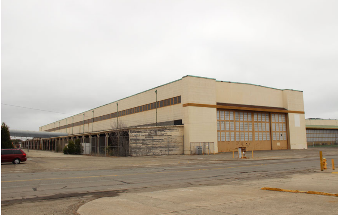
Figure 6. Building 9; view toward southeast.
