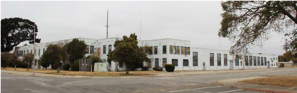
Figure 8. Building 114; view toward northeast.
