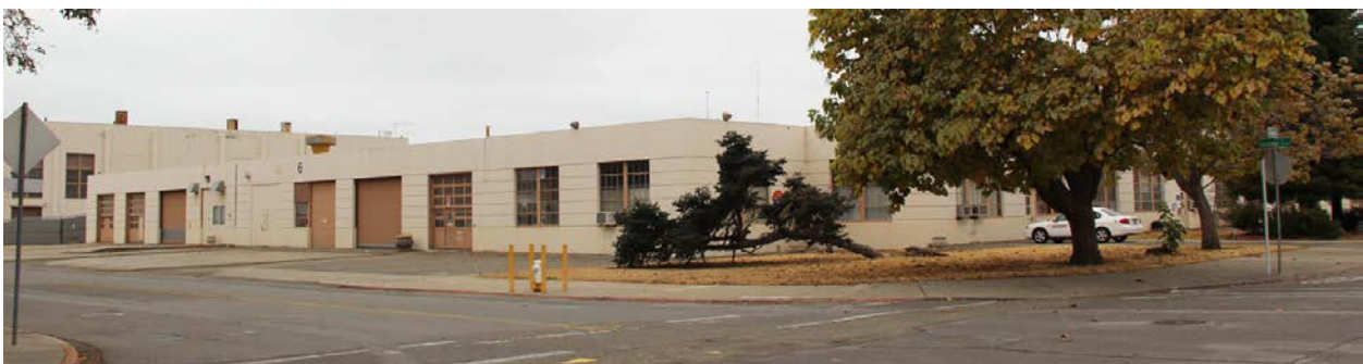
Figure 9. Building 6; view toward southwest.
