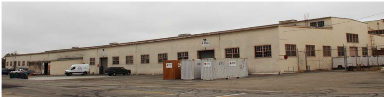
Figure 7. Building 92; view toward southeast.
