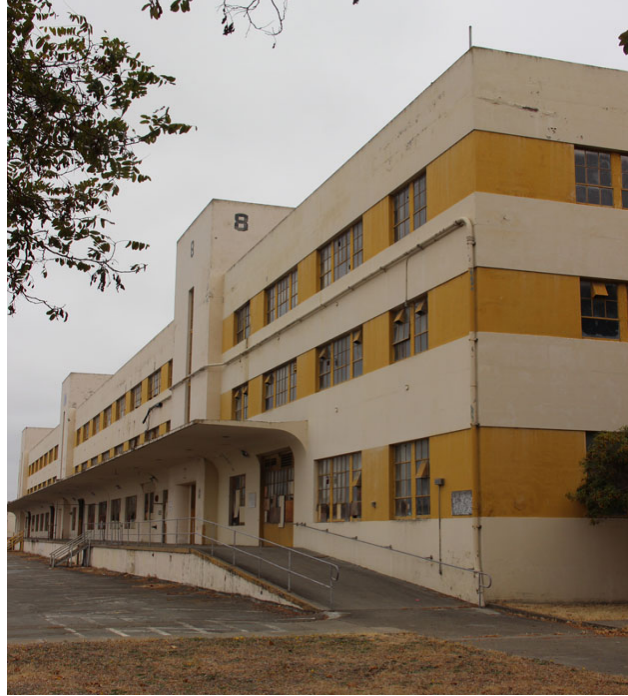
Figure 13. Loading dock on north façade of Building 8; view toward east.
