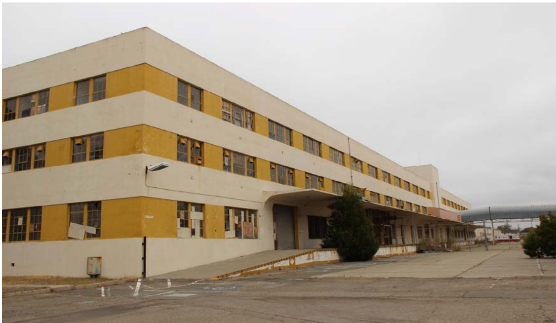
Figure 11. South façade of Building 8; view toward northeast.
