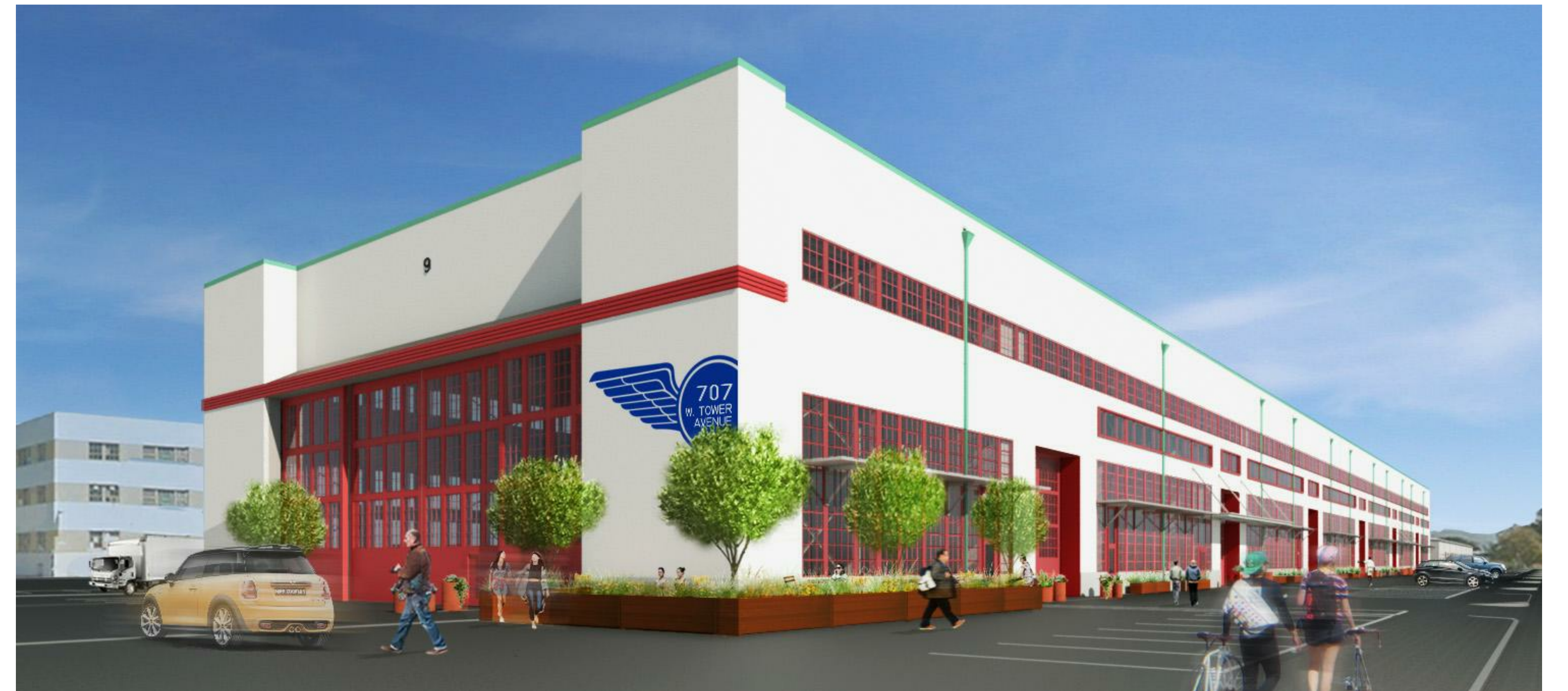
2 VIEW OF SOUTHWEST APPROACH
