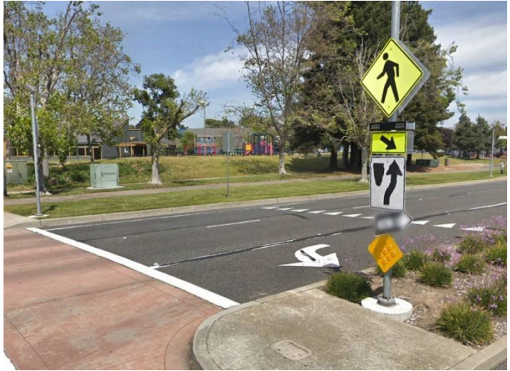
Figure 19: Pedestrian Crossing with an RRFB at the Intersection of Mecartney Road and Belmont Place on Bay Farm Island
