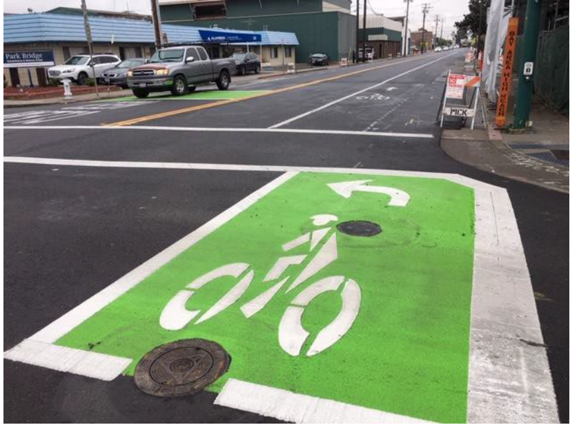
Figure 11. Two-stage left turn box located at the Park Street and Blanding Avenue intersection.
