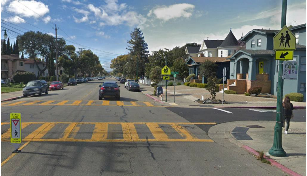
Figure 21: Streetside and In-Street Pedestrian Warning Signage at the Intersection of Santa Clara Avenue and Willow Street
