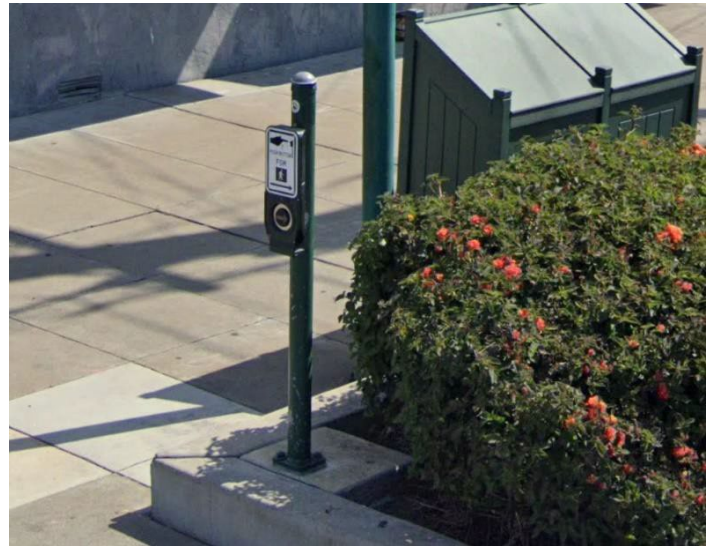
Figure 22: Audible Pedestrian Pushbutton at the Intersection of Webster Street and Lincoln Avenue
