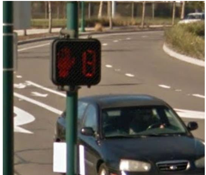
Figure 24: Pedestrian Countdown Signal at the Intersection of Willie Stargell Avenue and Webster Street
