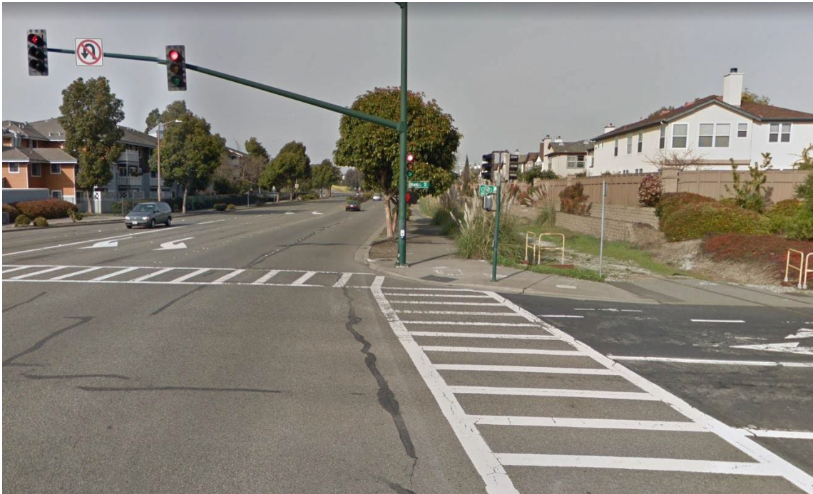
Figure 18: Ladder Style Crosswalks located at the Intersection of Constitution Way and Atlantic Avenue
