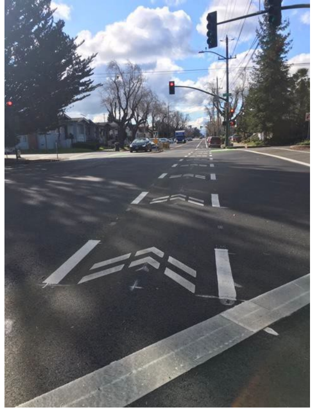
Figure 9. Bike lane extensions, using painted white dashed lines and chevrons, at the intersection of Tilden Way and Broadway.
