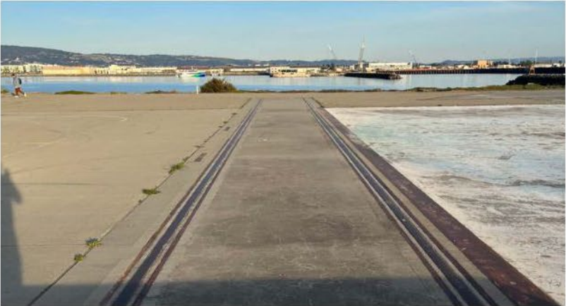
Rails Embedded in Concrete
