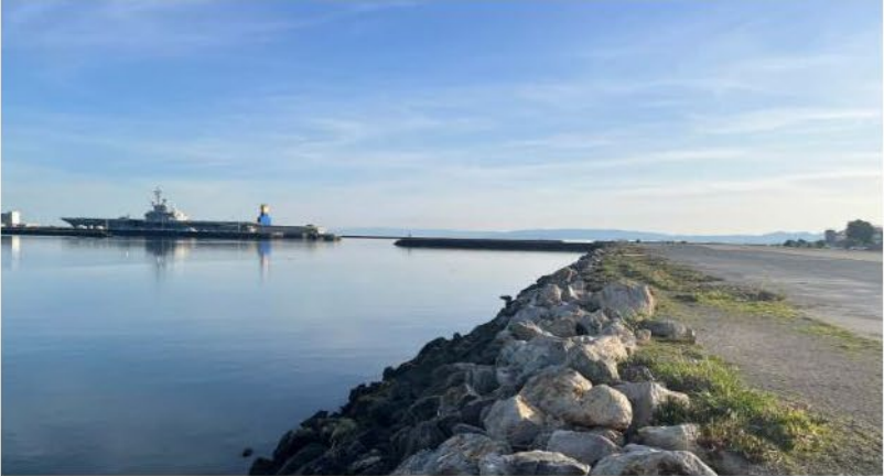
Seaplane Lagoon Armored Shoreline
