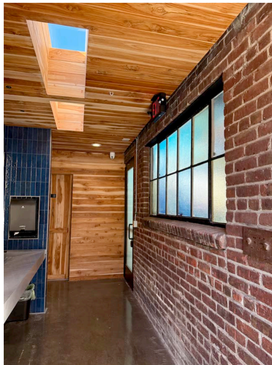
BREEZEWAY AT HANDWASH STATION
