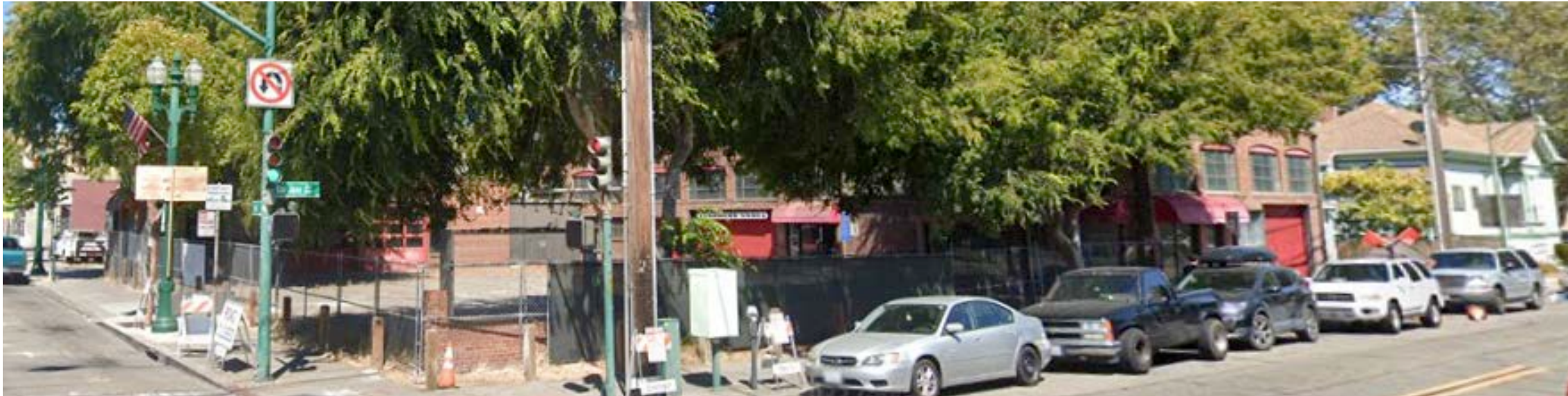
PRIOR TO START OF CONSTRUCTION
