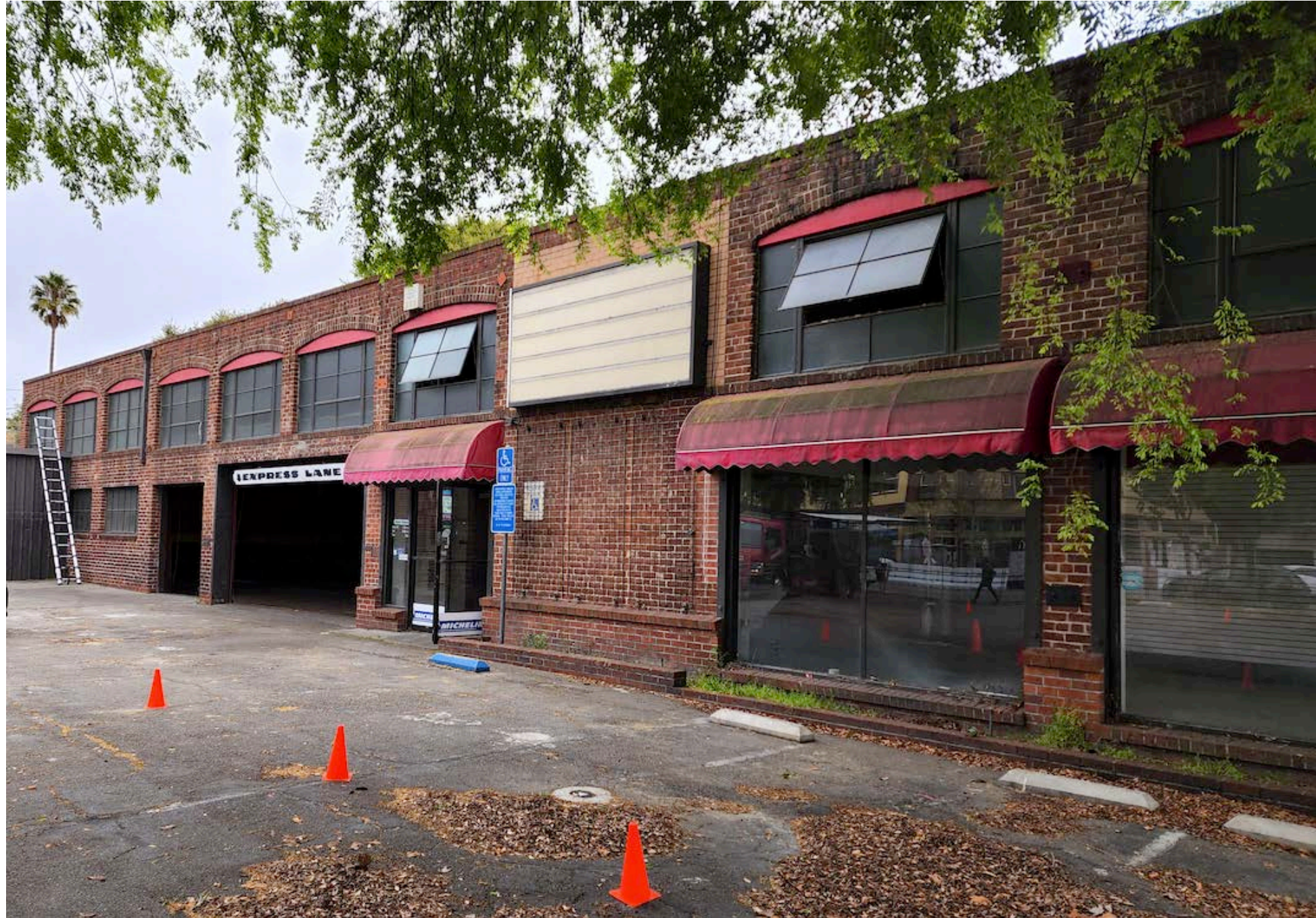
West elevation (looking North)
