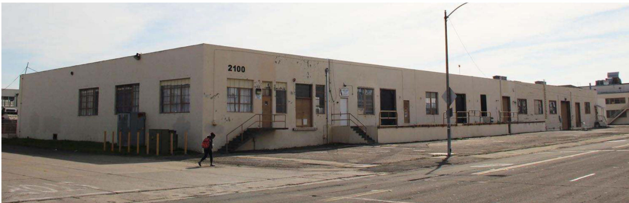
Figure 10. Building 13, looking southeast from the intersection of West Trident Avenue and Ferry Point Street Source: Christopher VerPlanck
