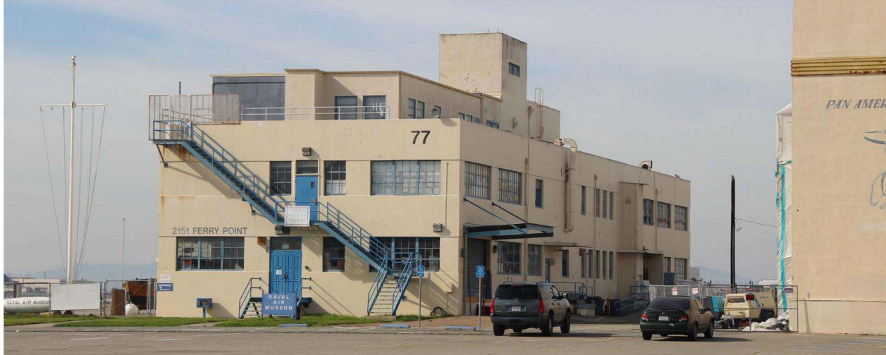
Figure 16. Building 77, looking southwest from the parking lot located to the east of Buildings 41 and 77 Source: Christopher VerPlanck
