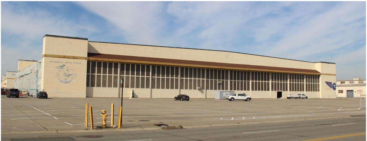
Figure 13. Building 41, looking northwest from Ferry Point Street Source: Christopher VerPlanck
