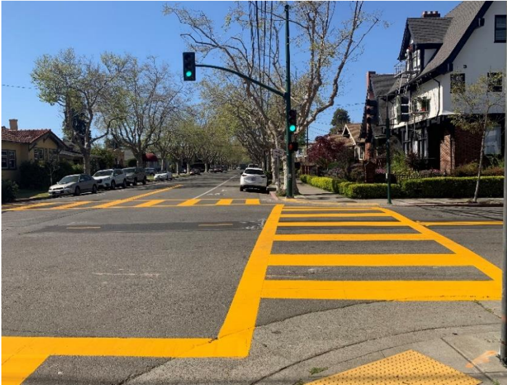
High-visibility crosswalks on Central Avenue
