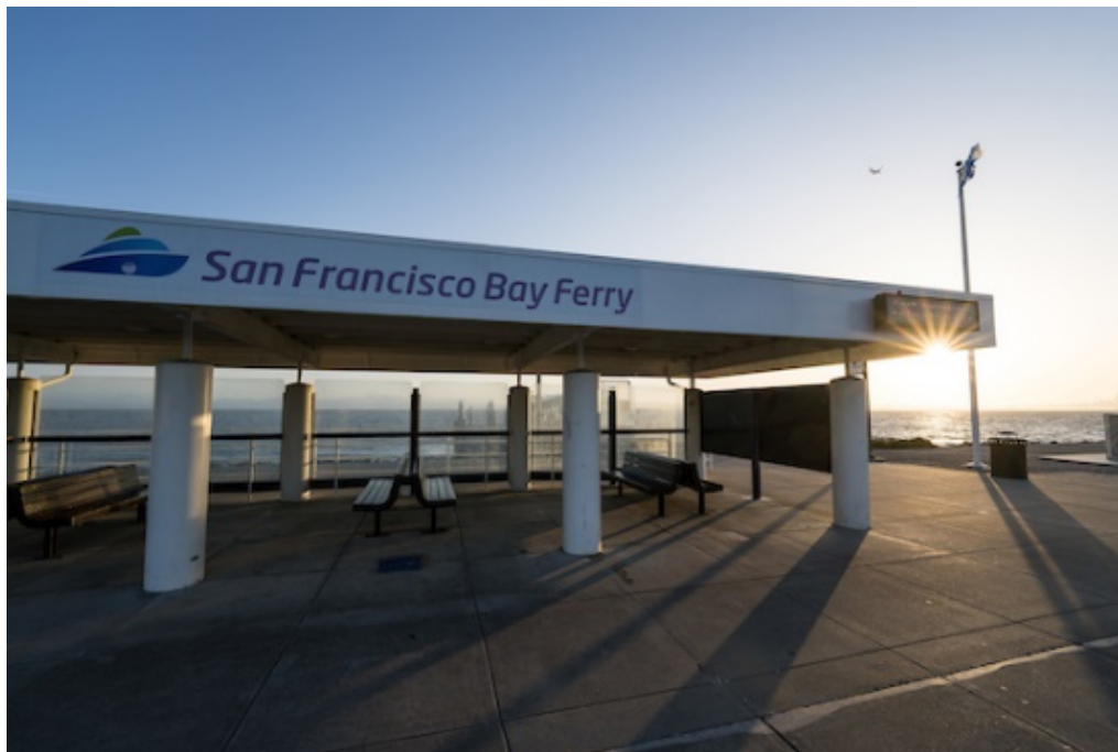
Figure 2: Harbor Bay Ferry Terminal
