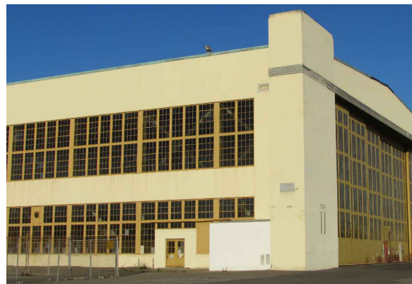
TOWER ELEMENT AND GLAZING
