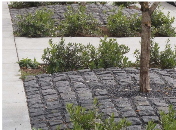
STONE COBBLES AT TREE WELLS
