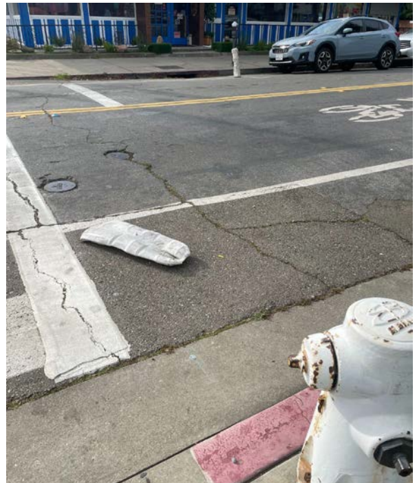
Author's photo of a fallen quick-build bollard, taken in Alameda in January 2022, shows the importance of including maintenance in Rapid Response planning
