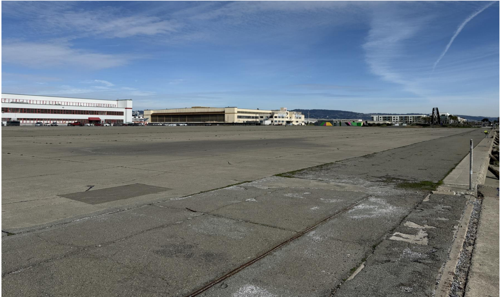
Taxiway, viewed from Seaplane Ramp No. 3, facing NE – Feb 2026 (J. Bevan)
