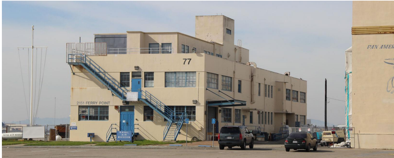
Figure 16. Building 77, looking southwest from the parking lot located to the east of Buildings 41 and 77 Source: Christopher VerPlanck
