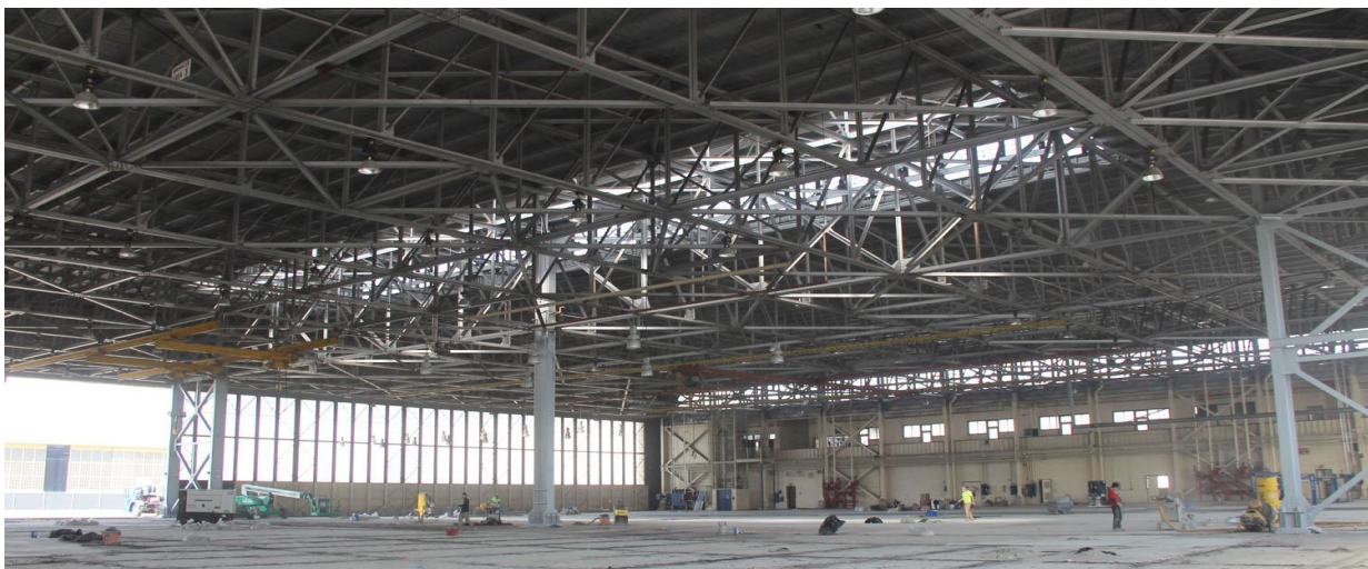
Figure 14. Building 41 interior, looking northwest Source: Christopher VerPlanck
