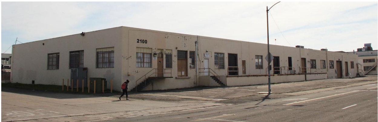
Figure 10. Building 13, looking southeast from the intersection of West Trident Avenue and Ferry Point Street Source: Christopher VerPlanck
