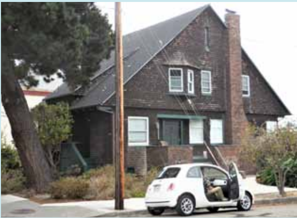
2000 Clinton prior to exterior restoration.
