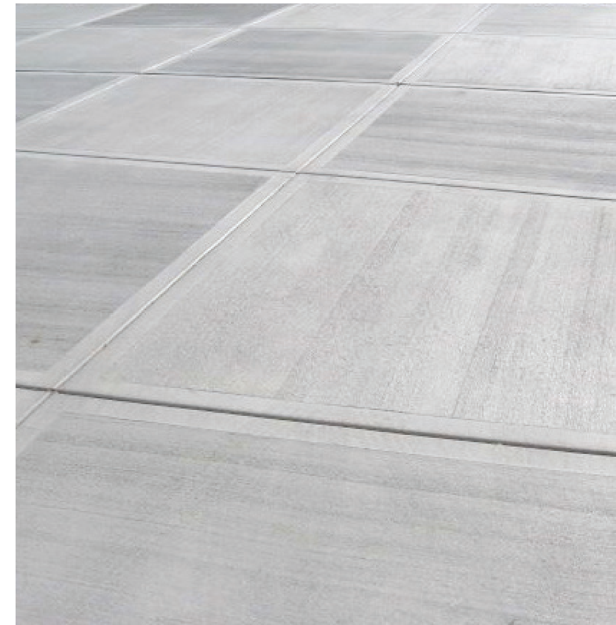
Broom Finish Concrete Sidewalks
