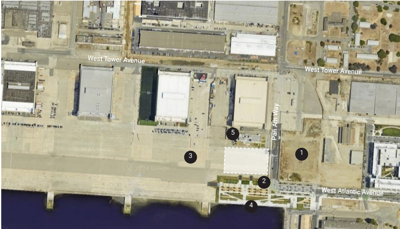
AERIAL VIEW OF SITE
