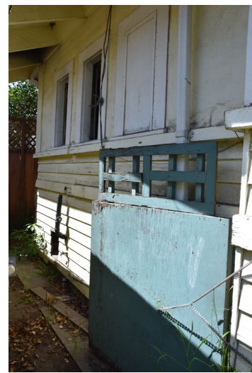
Figure 7. Oblique view of east façade, southern portion view southwest.
