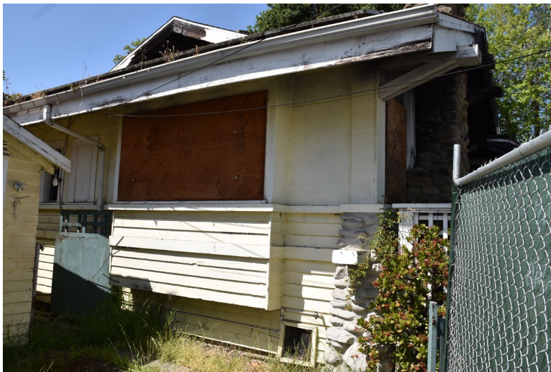
Figure 6. Oblique view of the east façade, northern portion, view southwest.
