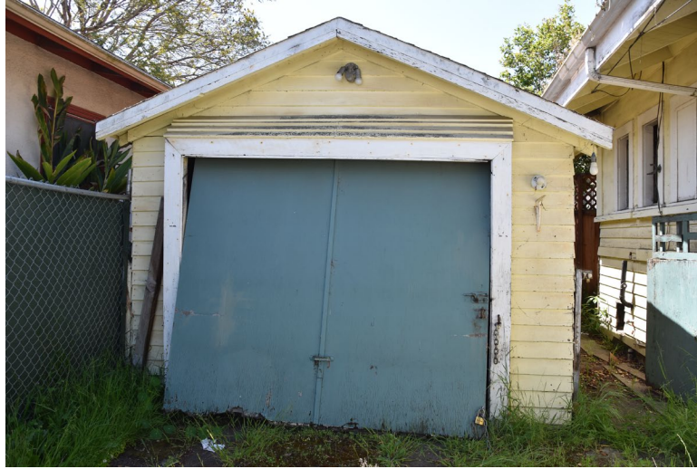
Figure 8. Garage, north façade, view south.
