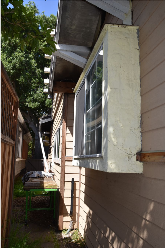
Figure 4. Oblique view of the rear south façade, view west.
