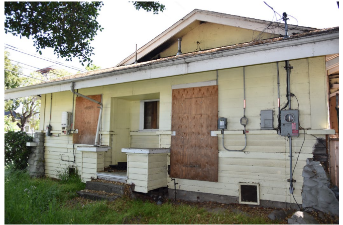
Figure 3. Oblique view of the west façade, view northeast.
