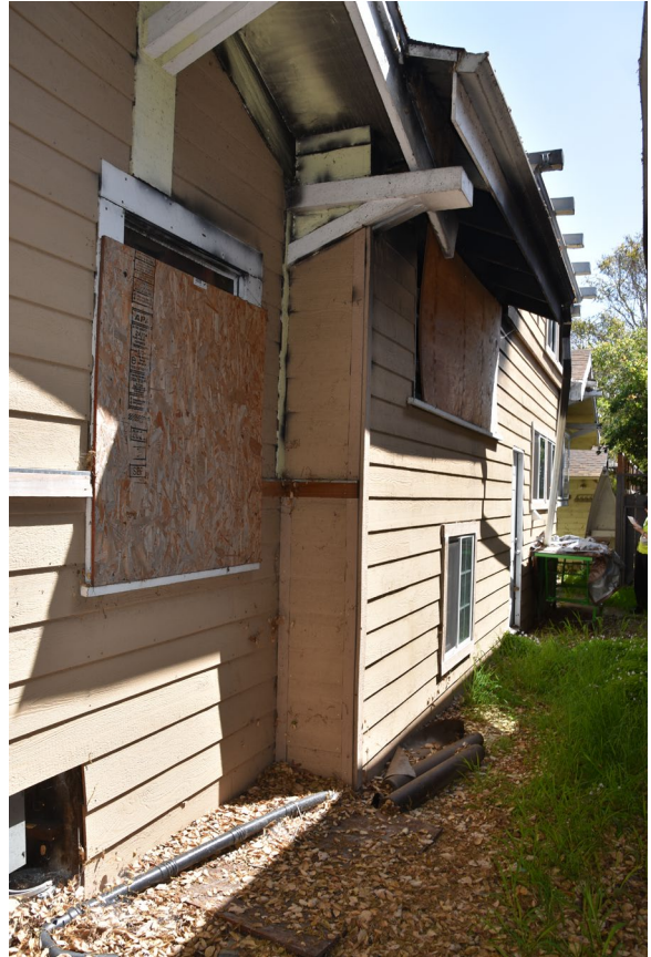
Figure 5. Oblique view of the rear south façade and bay, view east.
