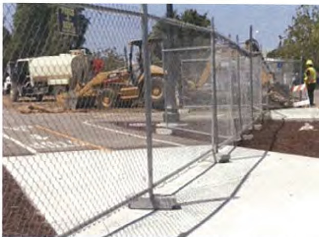
Construction on Alameda's Jean Sweeney CAT Trail Crossing.
