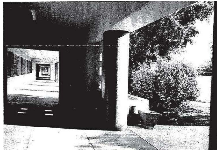
OVAL COLUMNS ARCADE IN BUILDING 2
