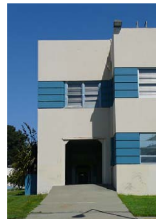
HORIZONTAL CONCRETE BANDS AND QUOIN ELEMENTS
