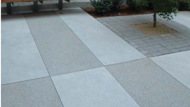
④ CONCRETE UNIT PAVERS AT SHARED PLAZA PARKING SPACES + ALL TREE WELLS
