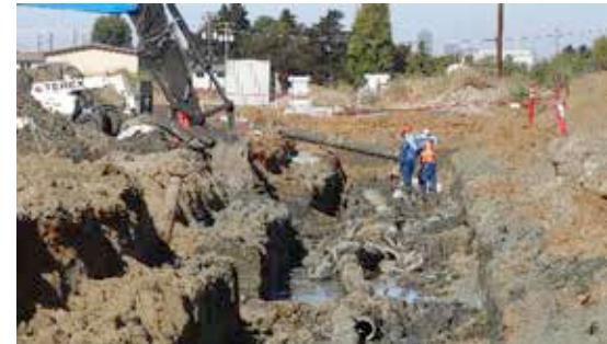
Utility Removal/Groundwater Extraction
