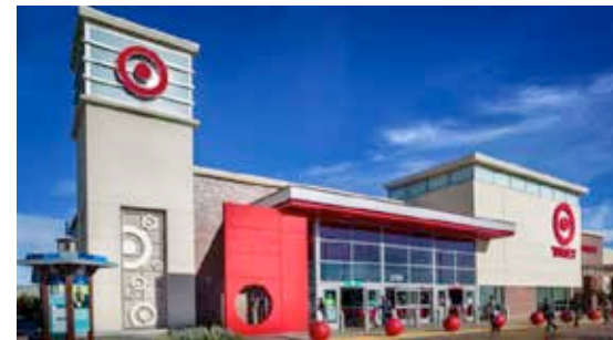
Completed Target Building (Pile Supported)
