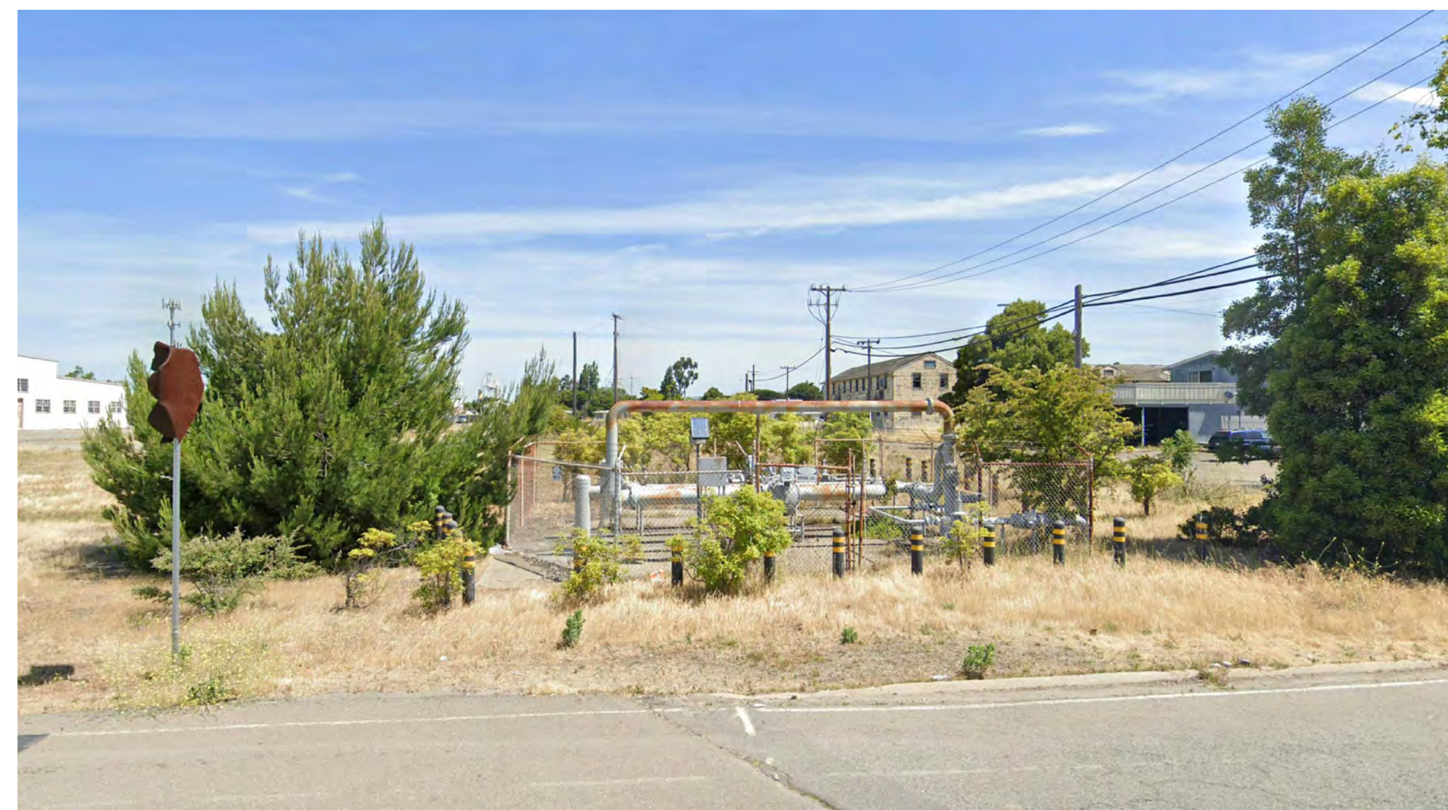
2. PG&E GAS FACILITY
