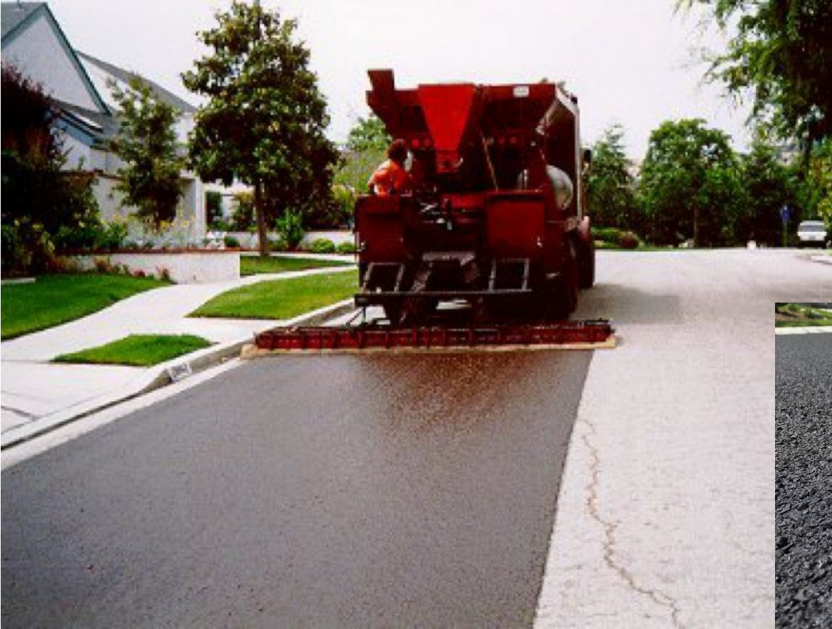
Slurry and Cape Seal
