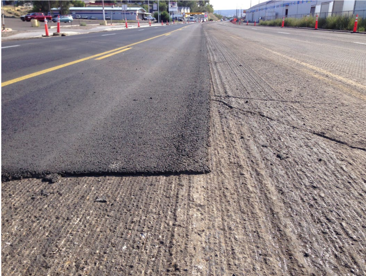
Traditional Overlay or Resurfacing
