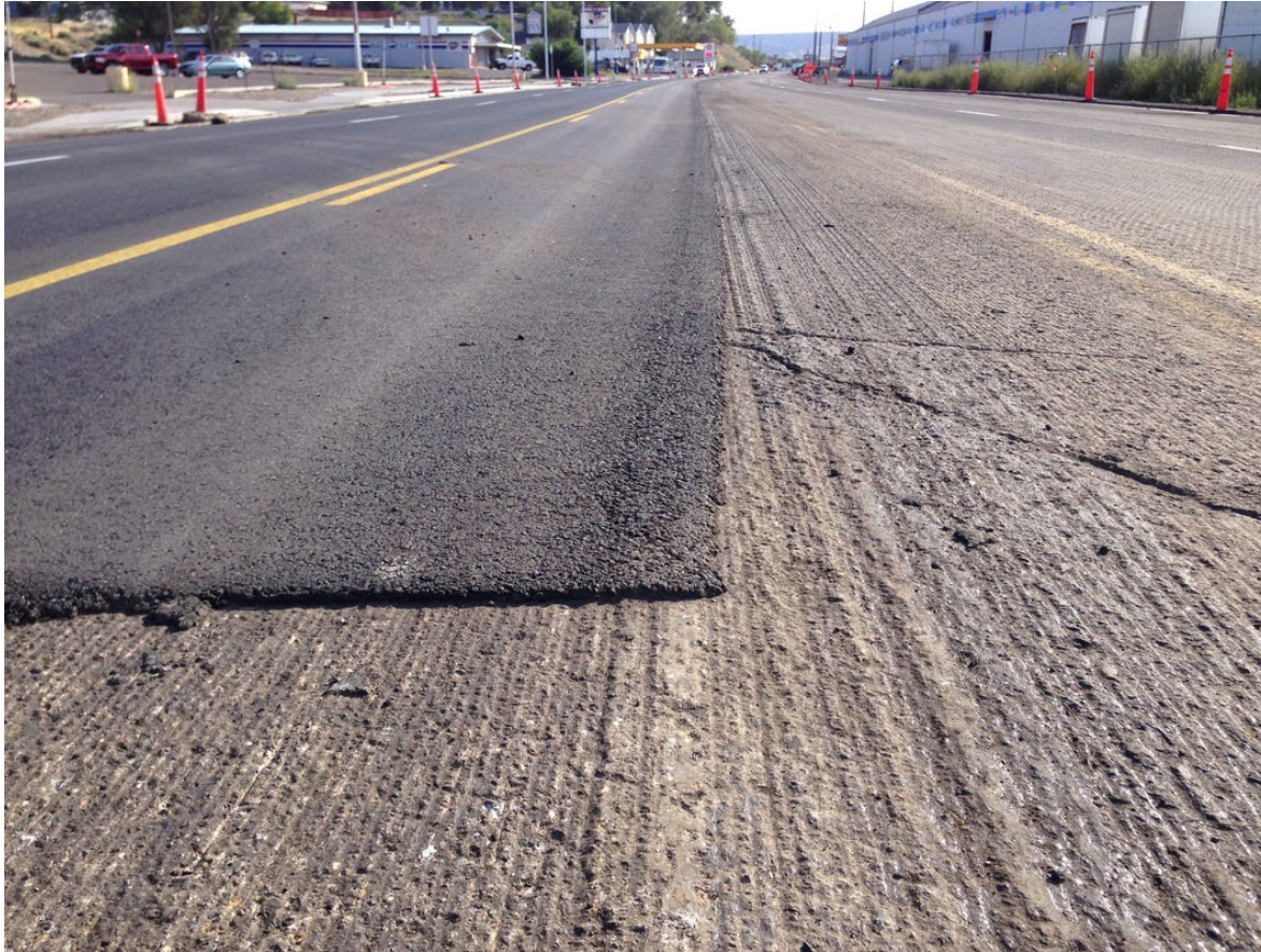
Traditional Overlay or Resurfacing
