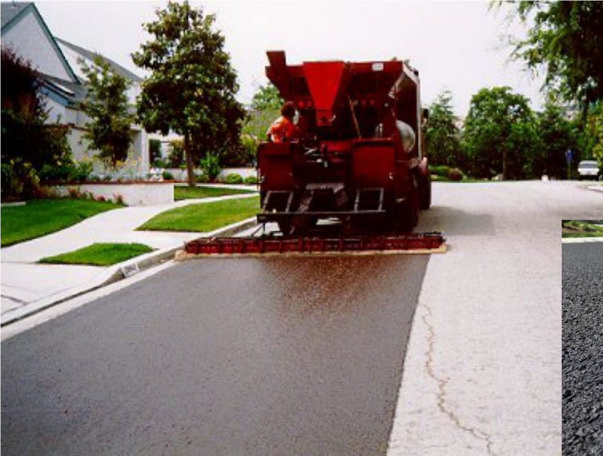
Slurry and Cape Seal
