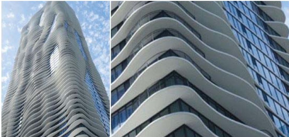
Louvres, Aqua Tower, Chicago
