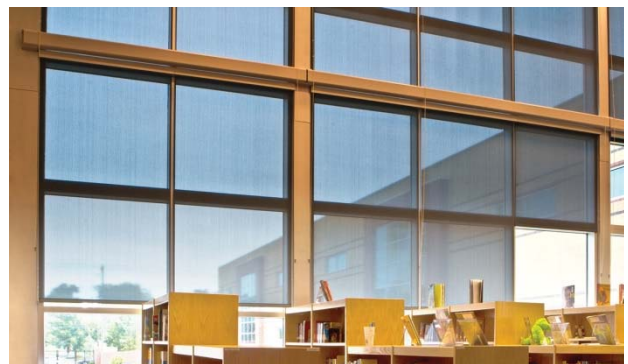
Solar blinds as seen from interior of a library.
