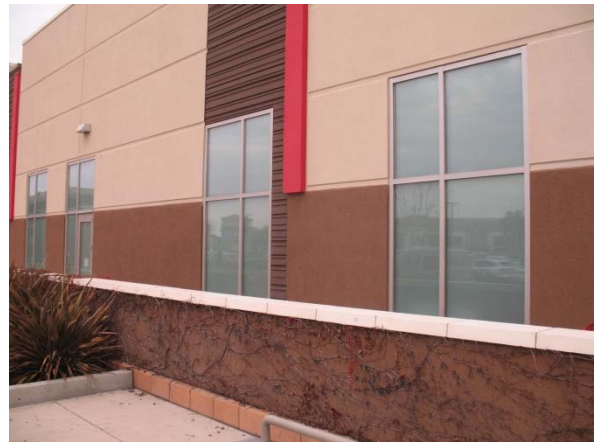
Translucent windows, Target store, Alameda.
