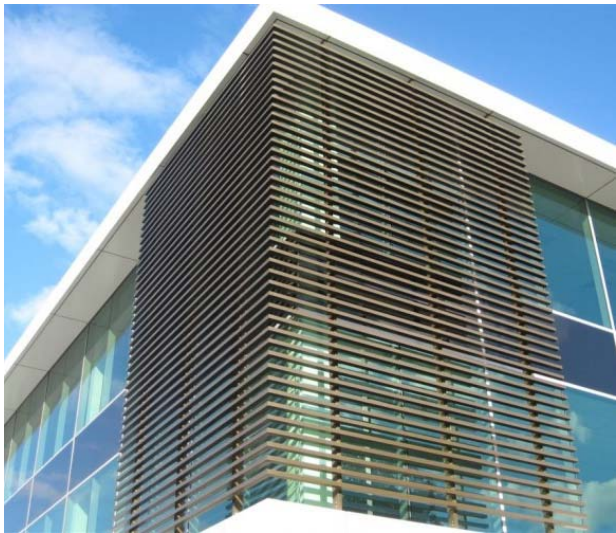
Louvres, Bayside Business Park, Queensland, Australia.
