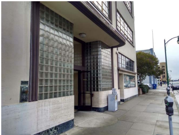
Glass block at first floor of commercial building across from Alameda City Hall.
