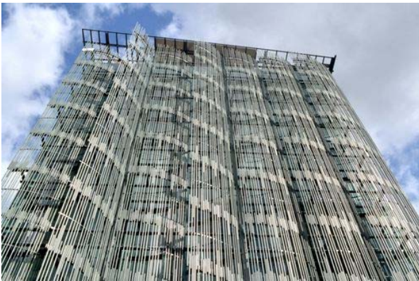
Screens, Edith Green – Wendell Wyatt Federal Building, Portland, OR.
