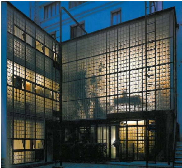
Modern building with glass block.
