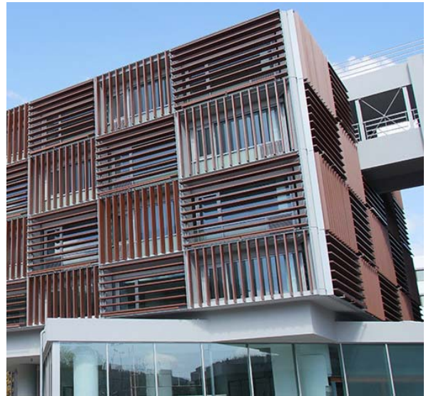
Louvres on renovated office building, by Glasscom.
