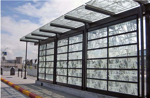
Bus stop with fritted glass, King County, Washington.
