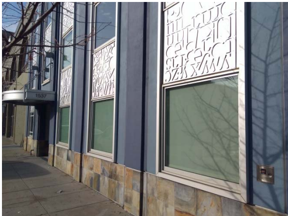
Interior screens on ground-floor windows, downtown Oakland.
