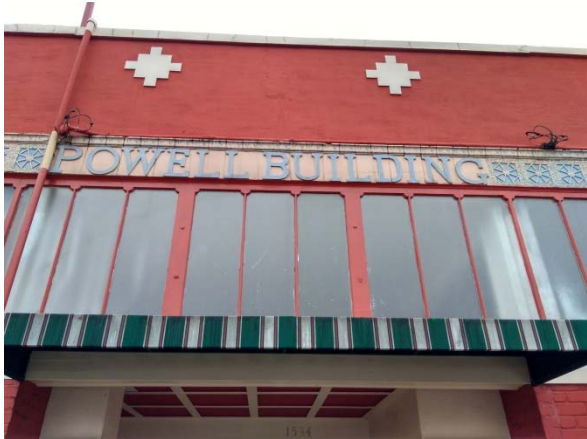
Translucent transom windows, Park Street, Alameda.
