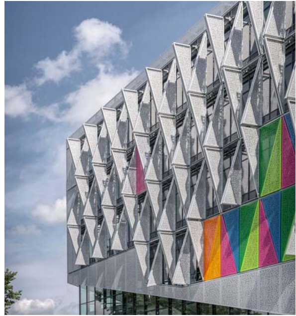
Sunshades, University of Southern Denmark
