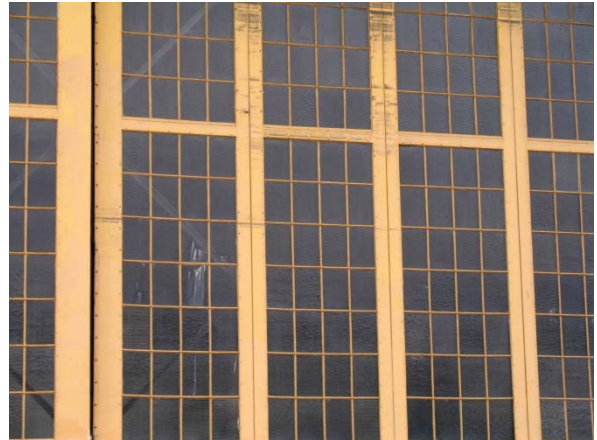
Steel sash windows in former hangar, Alameda Point.
