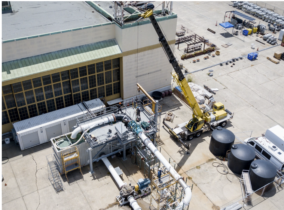
The equipment, pictured above, also includes some supporting water storage tanks (large black drums) that allow for the test system to be emptied and refilled when needed without unnecessarily wasting water. The position of these storage tanks will be to the west of the scale hydraulic test facility, obscuring them as much from public view behind the equipment while continuing to respect the boundaries of the USFWS Zone 1 (see Figure 6). These tanks are easily moved if necessary for Public Works sub-slab access.
